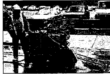
Correct PPE, but no control of sediments
