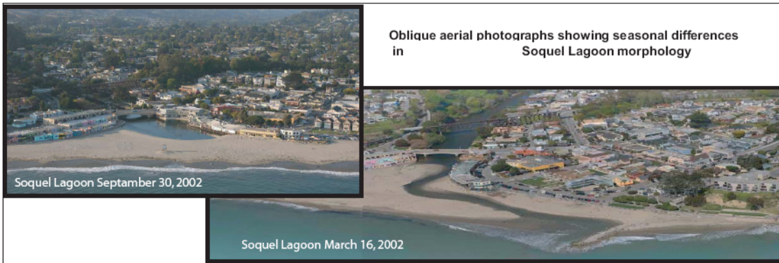
Figure 3: Photos of Soquel Lagoon (Swanson Hydrology)
