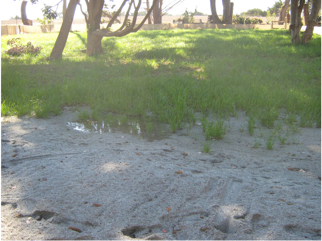
Ponded Effluent on Disposal Field 11-12-15
