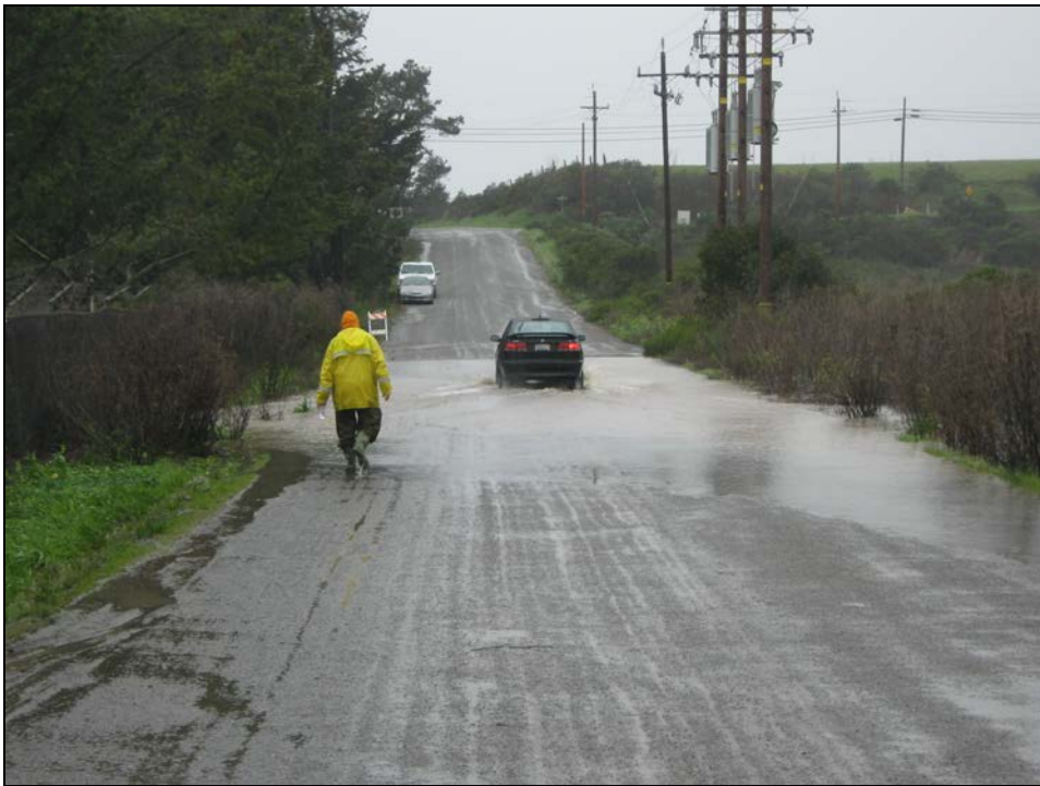
Storm water flowing across San Simeon Creek Rd. - February 17, 2017
