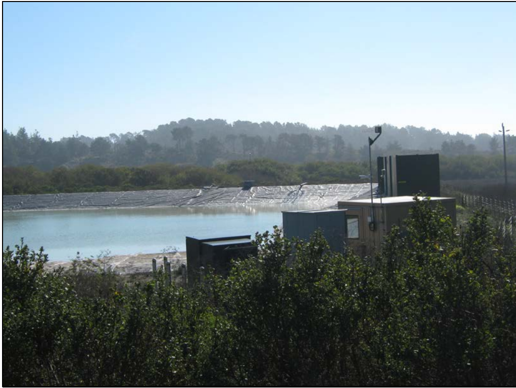
Impoundment water level - November 10, 2016
