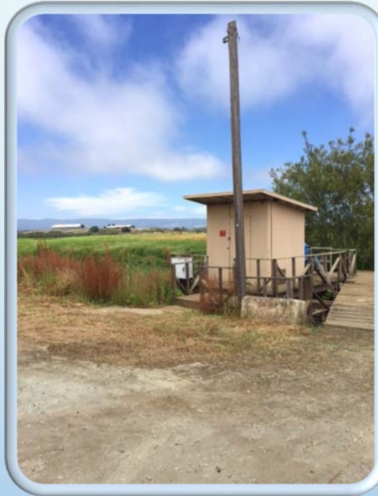
HARKINS SLOUGH DIVERSION
