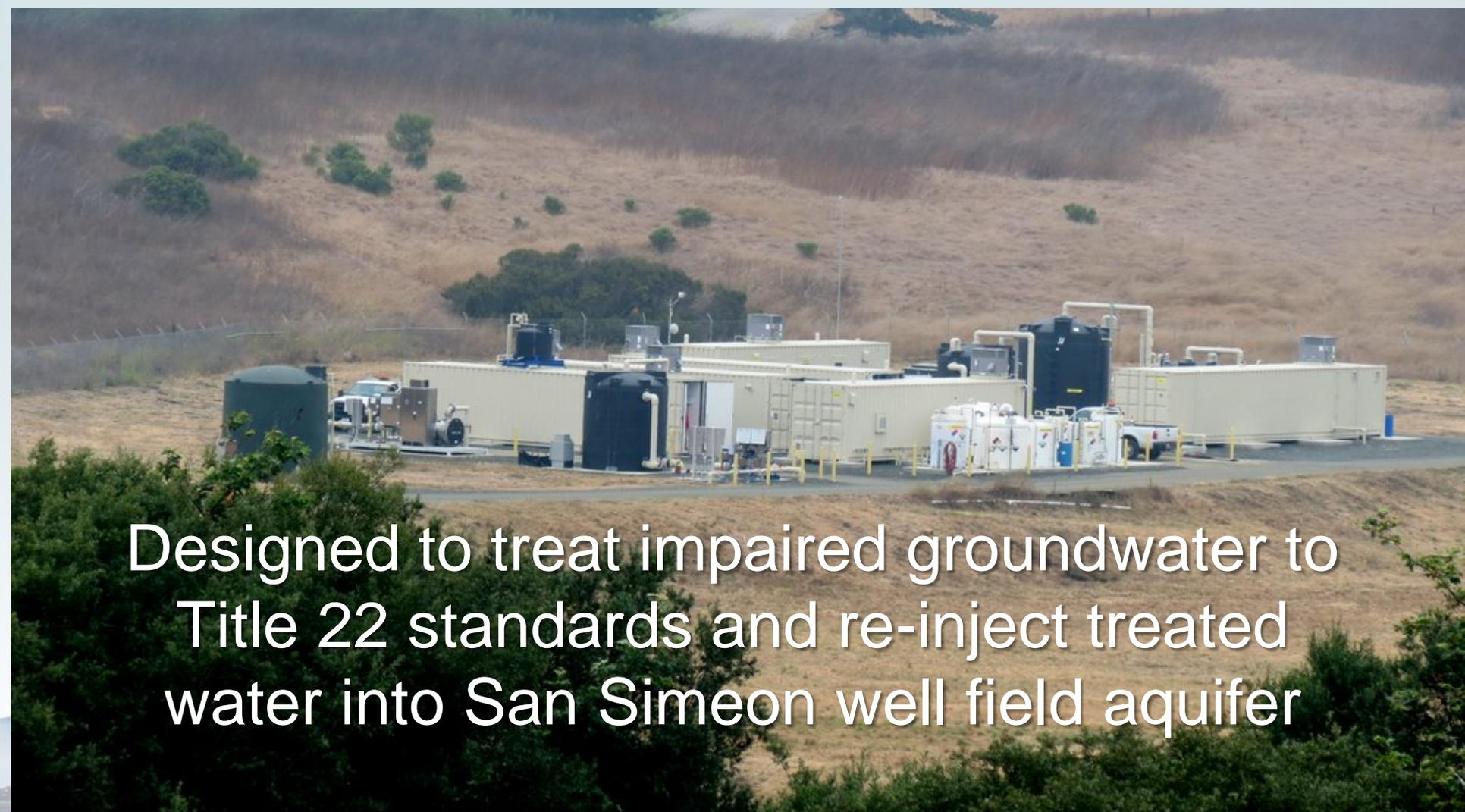
Designed to treat impaired groundwater to Title 22 standards and re-inject treated water into San Simeon well field aquifer
