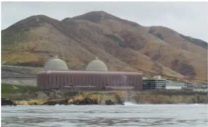
Diablo Canyon Nuclear Power Plant
