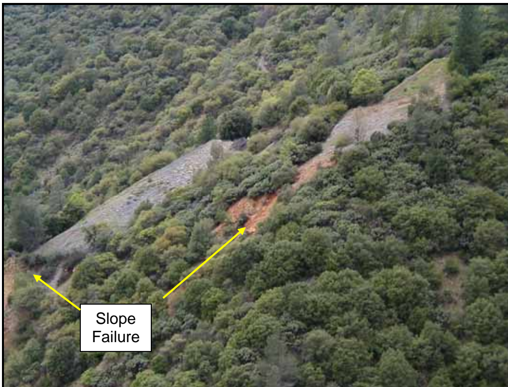
Photo 2. Slope Failures Waste Dumps #2 and #4.
