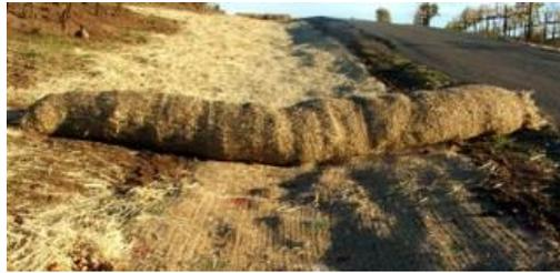
Figure 8: Wattles are used on slopes and in the avenues as standard practice.
