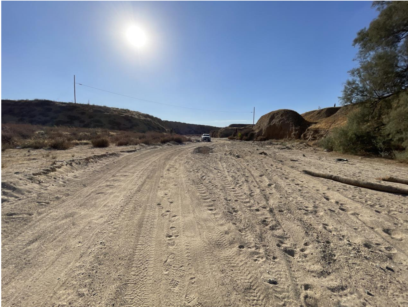
Photo 1: Upstream View of Sunset Avenue Crossing (Pershing Creek), Facing West
