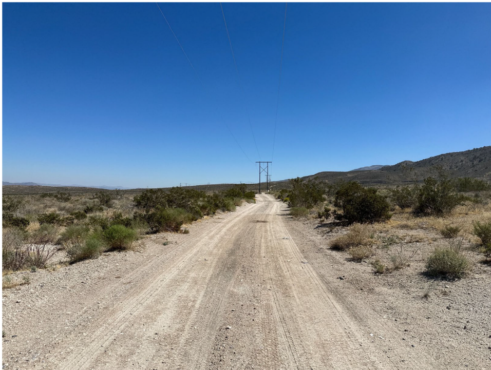
Photo 4. Existing Powerline Road, View Facing East
