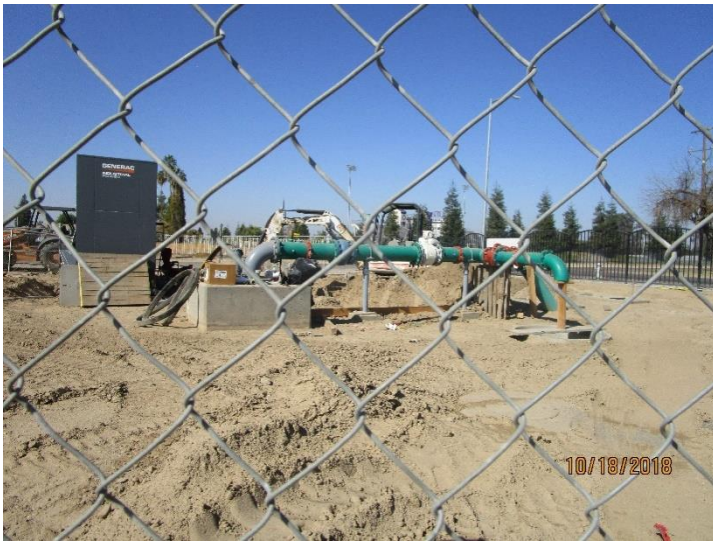
Figure 1. New well construction at WUHS
