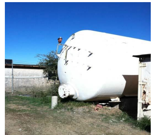
Substandard Water Tank
