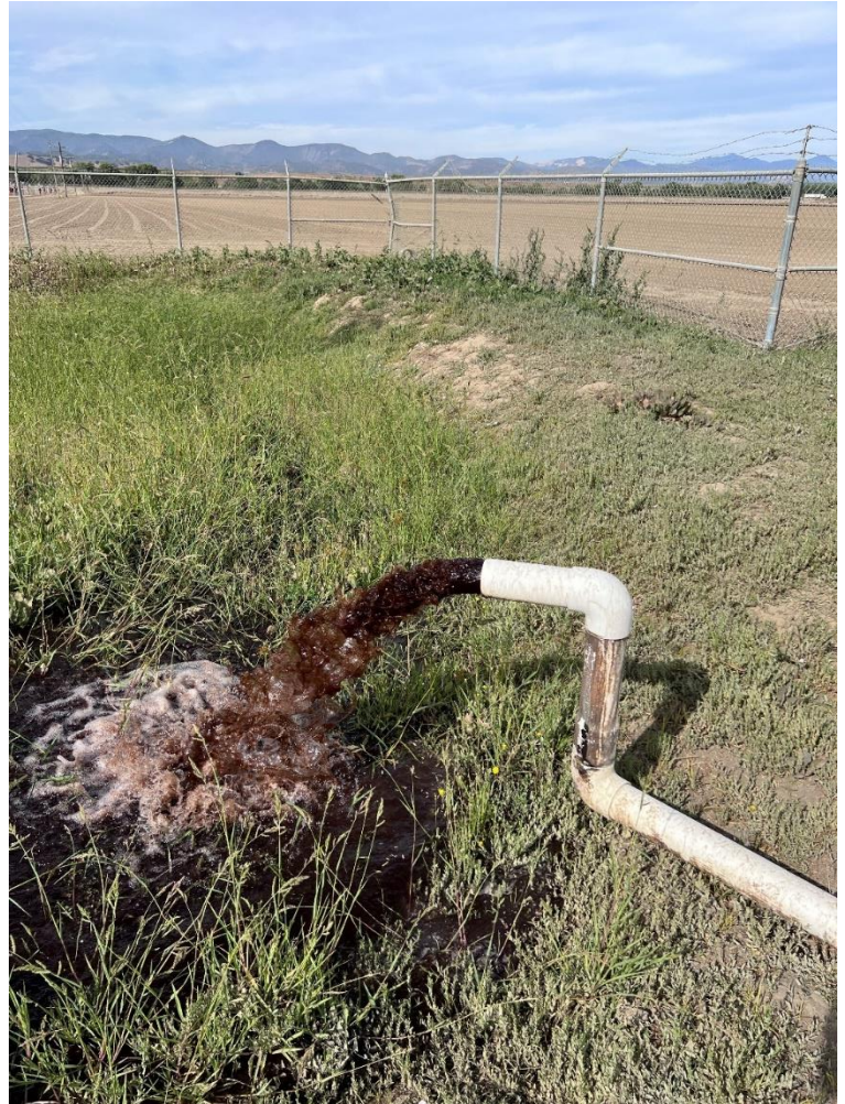
Wastewater from Filter Backwash
