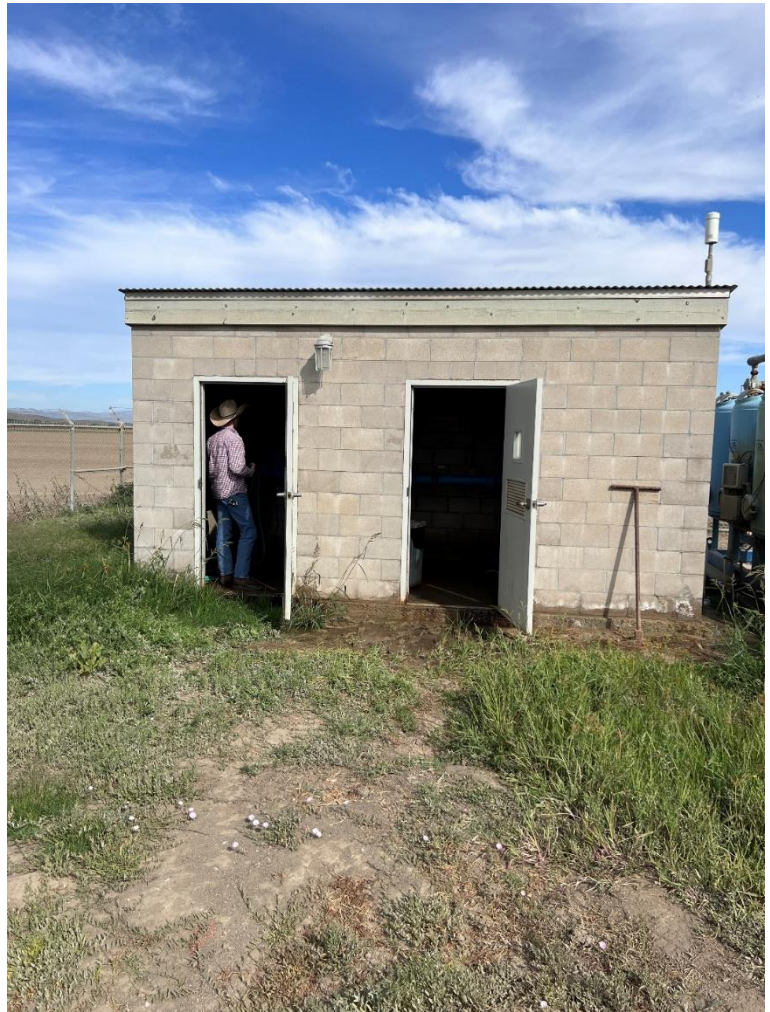
Chemical Storage/Injection Building
