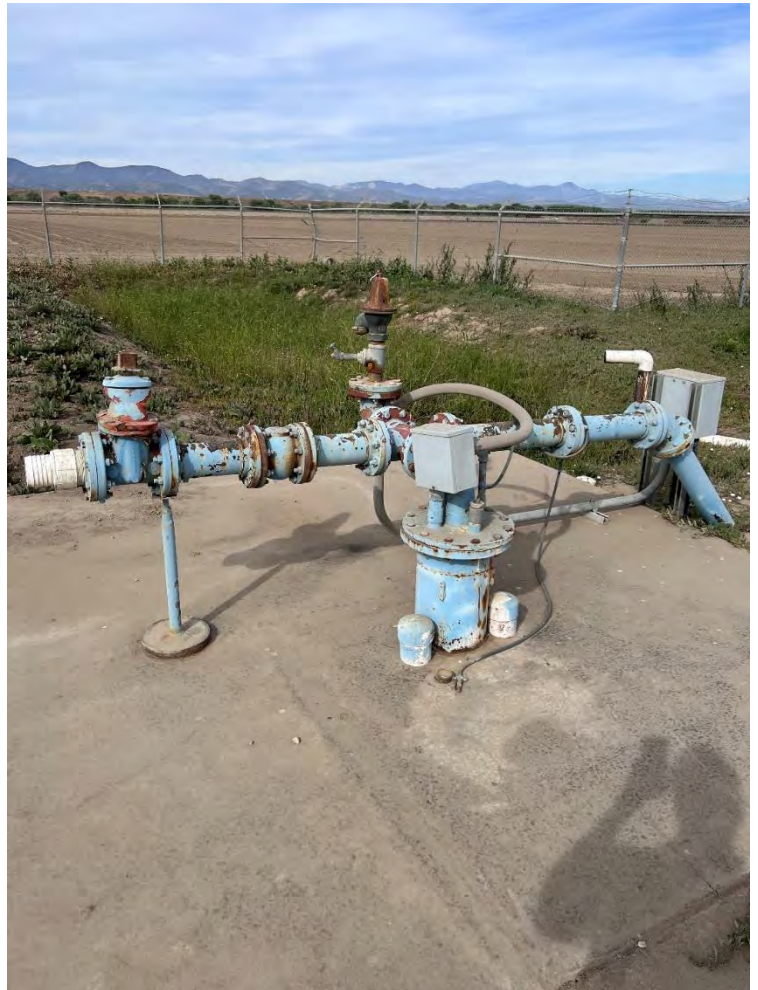
Abandoned Well at Treatment Facility
