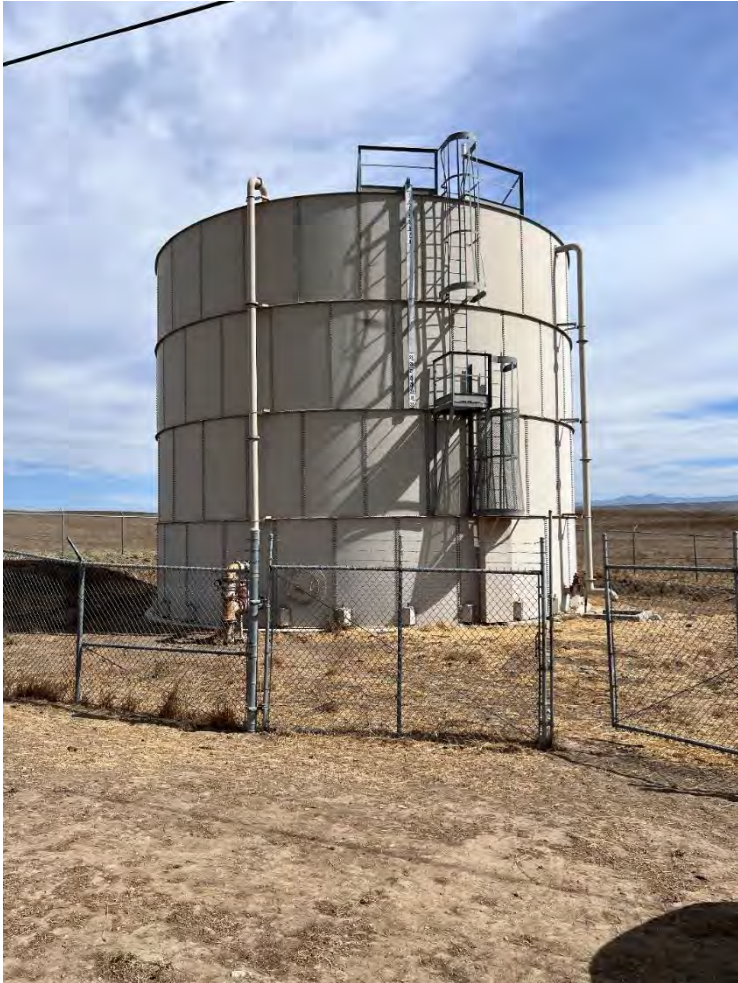
Overview of Storage Tank
