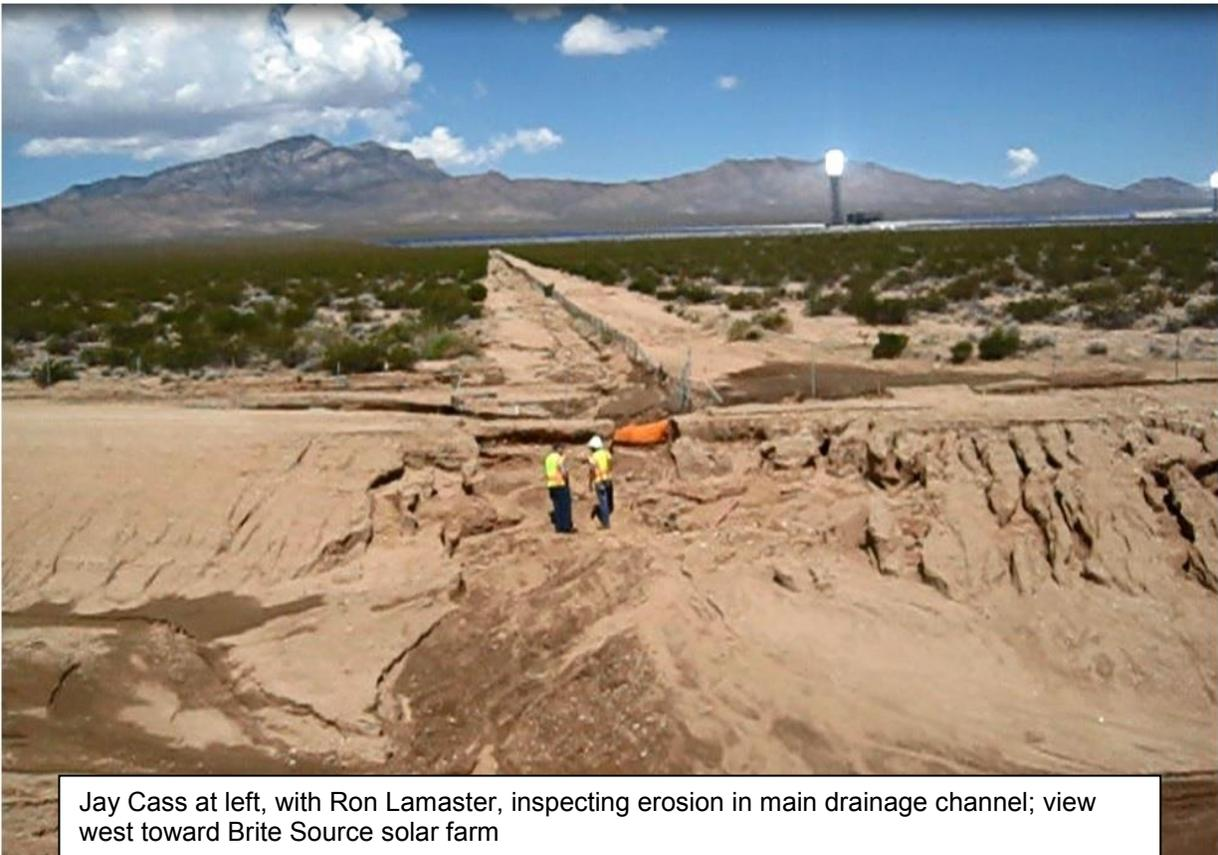
Jay Cass at left, with Ron Lamaster, inspecting erosion in main drainage channel; view west toward Brite Source solar farm
