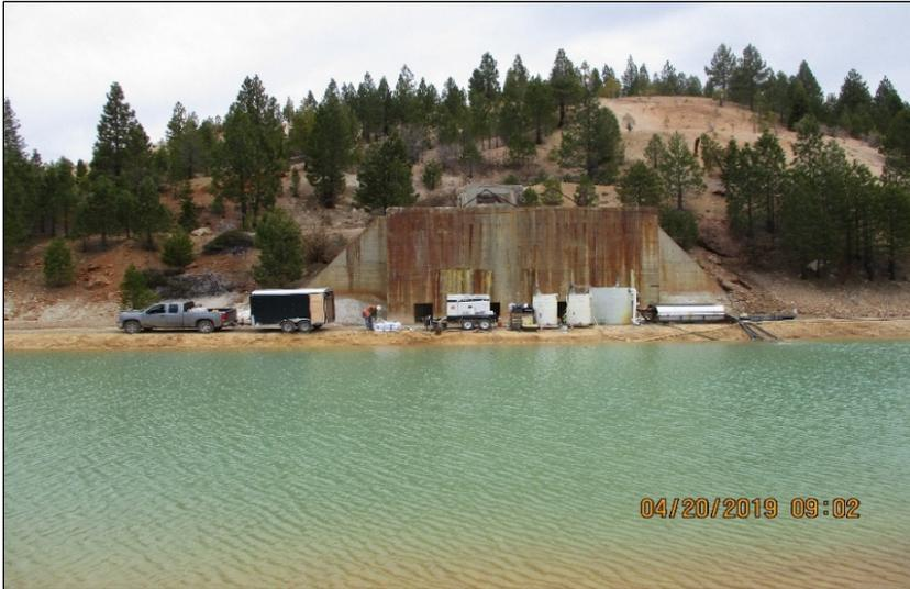
**Figure 3 - Pond 3 with Emergency Spring Treatment System, April 20, 2019**
