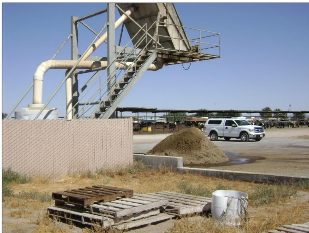
Figure 4.1: This machine, as a BMP, is used for separating manure solids from liquids. The liquids will be reused and applied as crop irrigation and fertilization water, increasing removal of nitrogen through crop uptake and decreasing nitrogen available for transport to groundwater.
