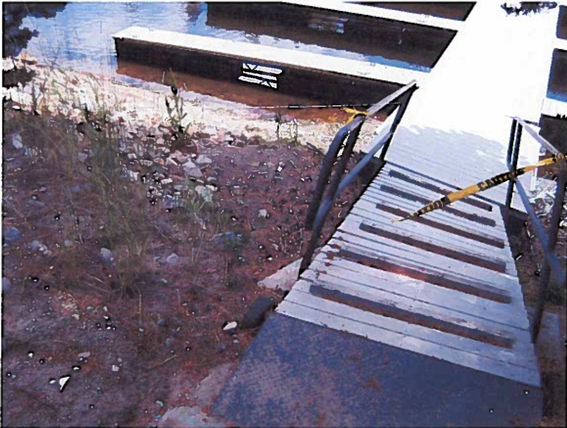
Photo 12 - Moving closer to the second ramp west of office to get a further close up within the marina area. Note that the fiber rolls were unable to prevent runoff from going down ramp and into marina, as evidenced by a sediment deposit in marina located on left (east) side of ramp.
