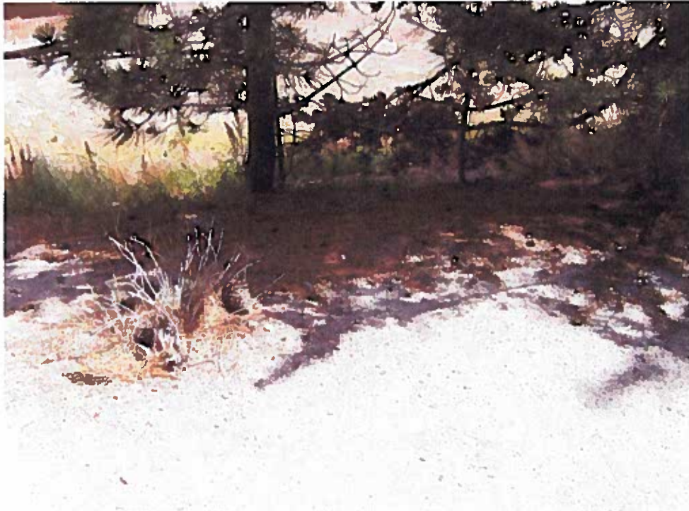
Photograph 29 - Standing at photo point 28, looking southwest. Fiber rolls have not been placed to collect potential stormwater runoff from the unpaved parking area.
