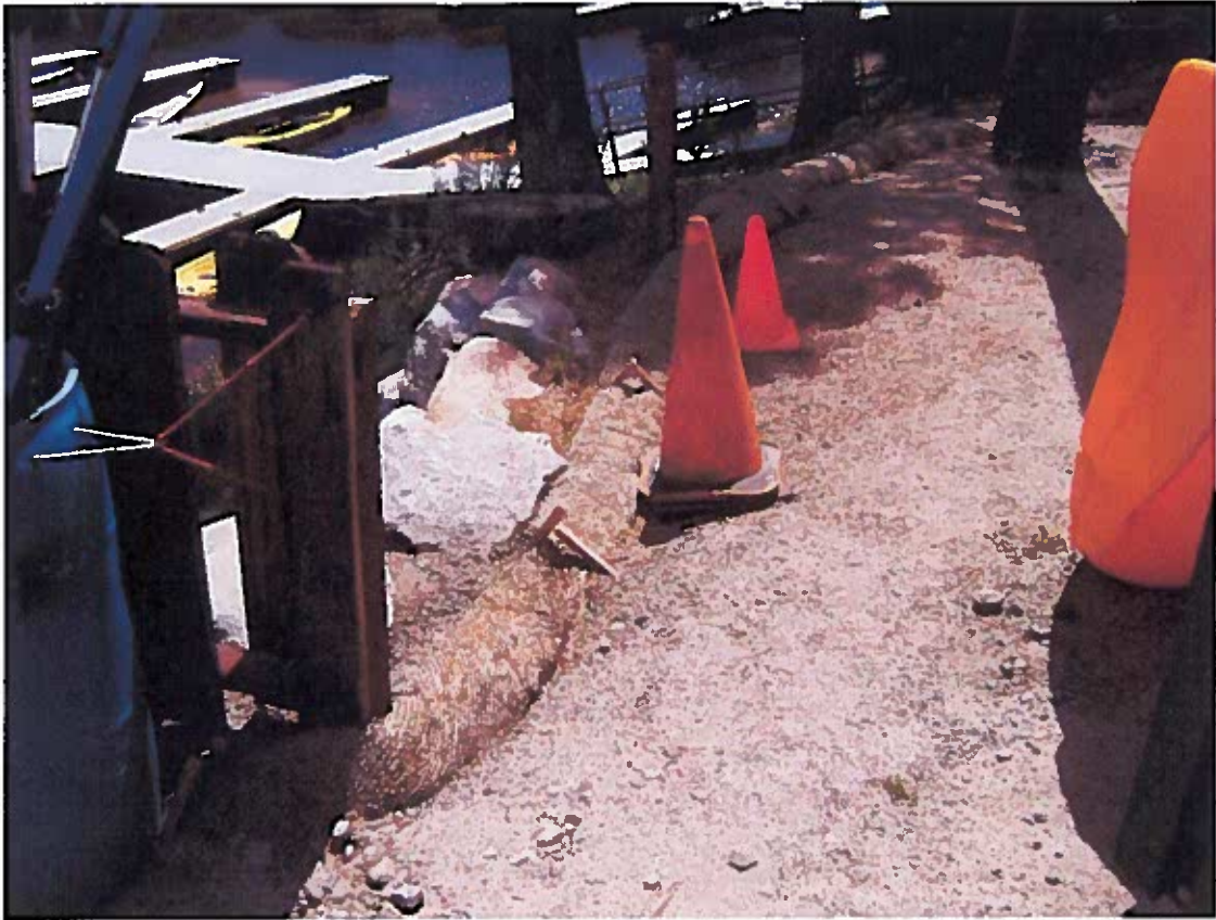
Photograph 05 - Flattened fiber roll adjacent to marina office, facing southwest. Also, the end of the fiber roll is installed perpendicular to the gradient, which will channelize storm water runoff.
