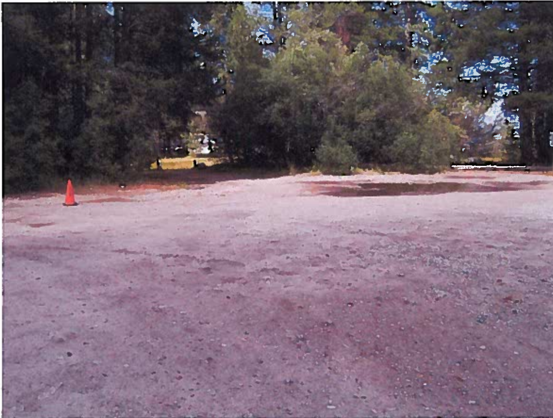
Photograph 03 - At Northeast area, Looking Northeast at Ponded Water In Parking Area. Per the SWPPP, the infiltration area should be located roughly where the willow stand in the center of the photograph is located. This Photograph was taken at the conclusion of the inspection at approximately 3:10 p.m.
