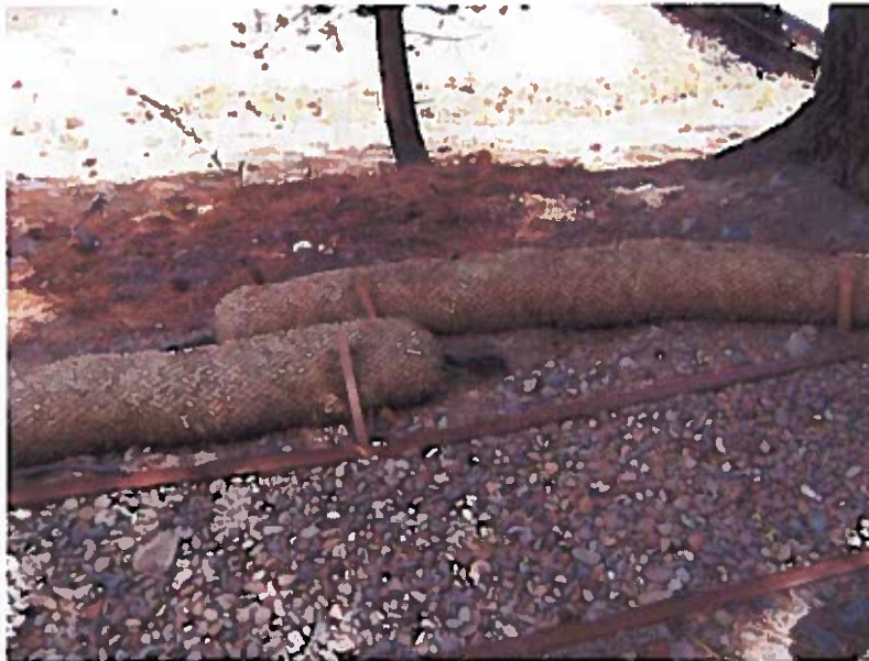
Photograph 19 - West of photo 18, between 3rd and 4th ramps west of office. In this area, the fiber rolls are adequately overlapped.
