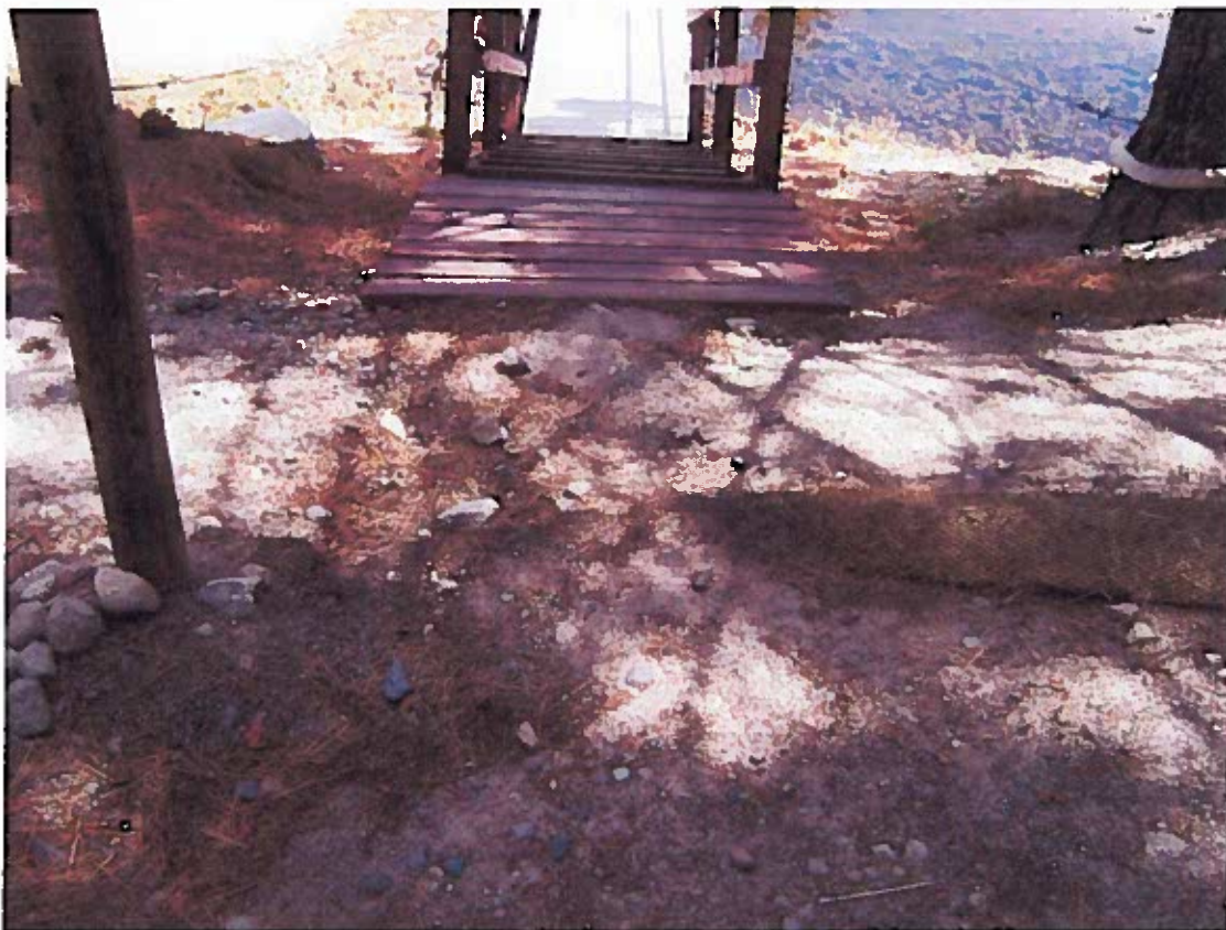
Photograph 22 - Close up of the sediment-inundated fiber roll shown in Photograph No. 20, also showing sediment deposits down along the embankment and into Lake Tahoe.
