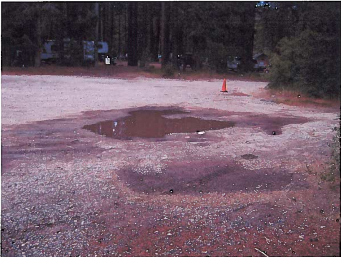
Photograph 02 - Facing West Toward Parking Area, Panning right of Photo 1, Standing Ponded Water in Lot From Recent Rains
