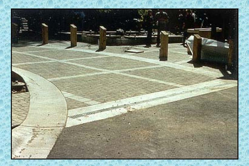
Permanent stormwater filtration systems like these can also be a good way to control pollutants in stormwater runoff.
