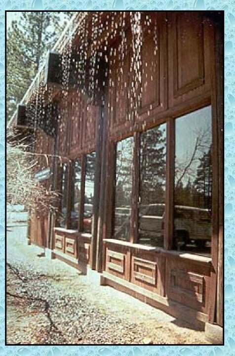
The gravel at the base of this structure handles roof runoff without using drains or gutters. The runoff infiltrates into the natural permeabile soil. (Lake Tahoe, CA) This permeable drainage system allows the runoff from this office building's parking lot to be reabsorbed into the ground, preventing pollution to surface water. (Lake Tahoe, CA)
