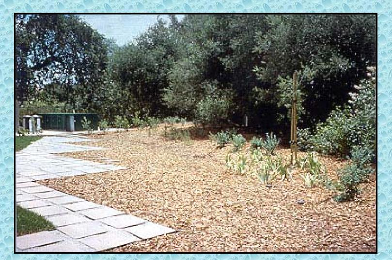
Unit paving on a sand bed allows infiltration of some runoff and reduces pollutants.
