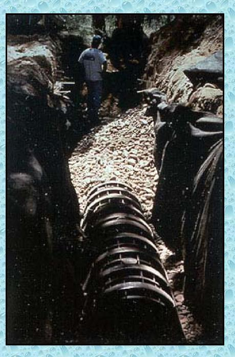
This gravel filtration system treats runoff so that pollutants are removed through soil media.
