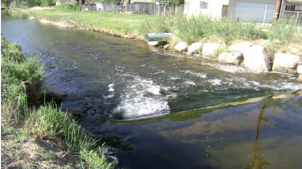
Photo 7-1 Concrete encased clay pipe submerged in water at a canal crossing. City of Bishop planned to replace this 15-inch clay pipe with a new 18-inch plastic pipe (more information contained in Section 7.5.3). Photo credit: John Morales/Lahontan Water Board
