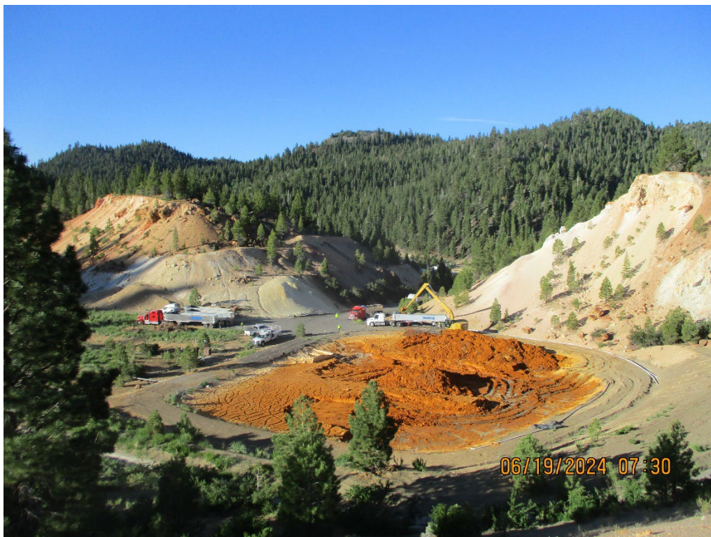
Photo 4 – June 19, 2024, Sludge removal and disposal activities at the Pit Clarifier. Approximately 2,025 tons of sludge was removed and disposed of.
