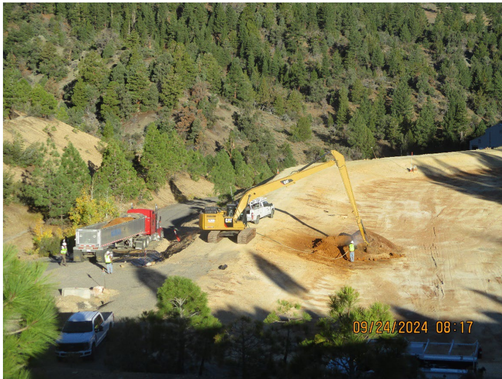
Photo 8 – September 24, 2024, Sludge haul activities at Pond 3. Approximately 88 tons of sludge was removed and disposed of.
