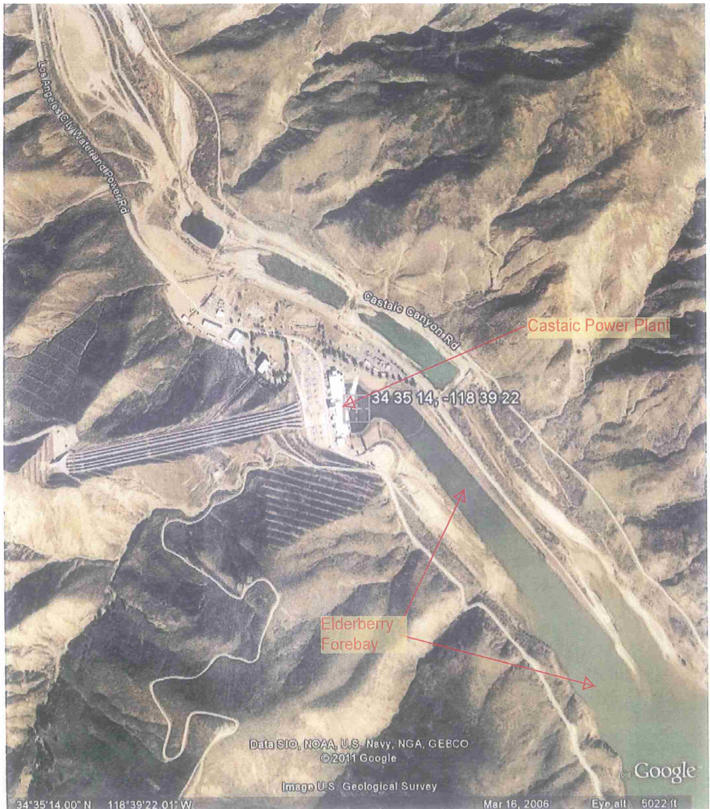
Aerial View Showing Castaic Power Plant and Elderberry Forebay. Approximate coordinates are shown.
