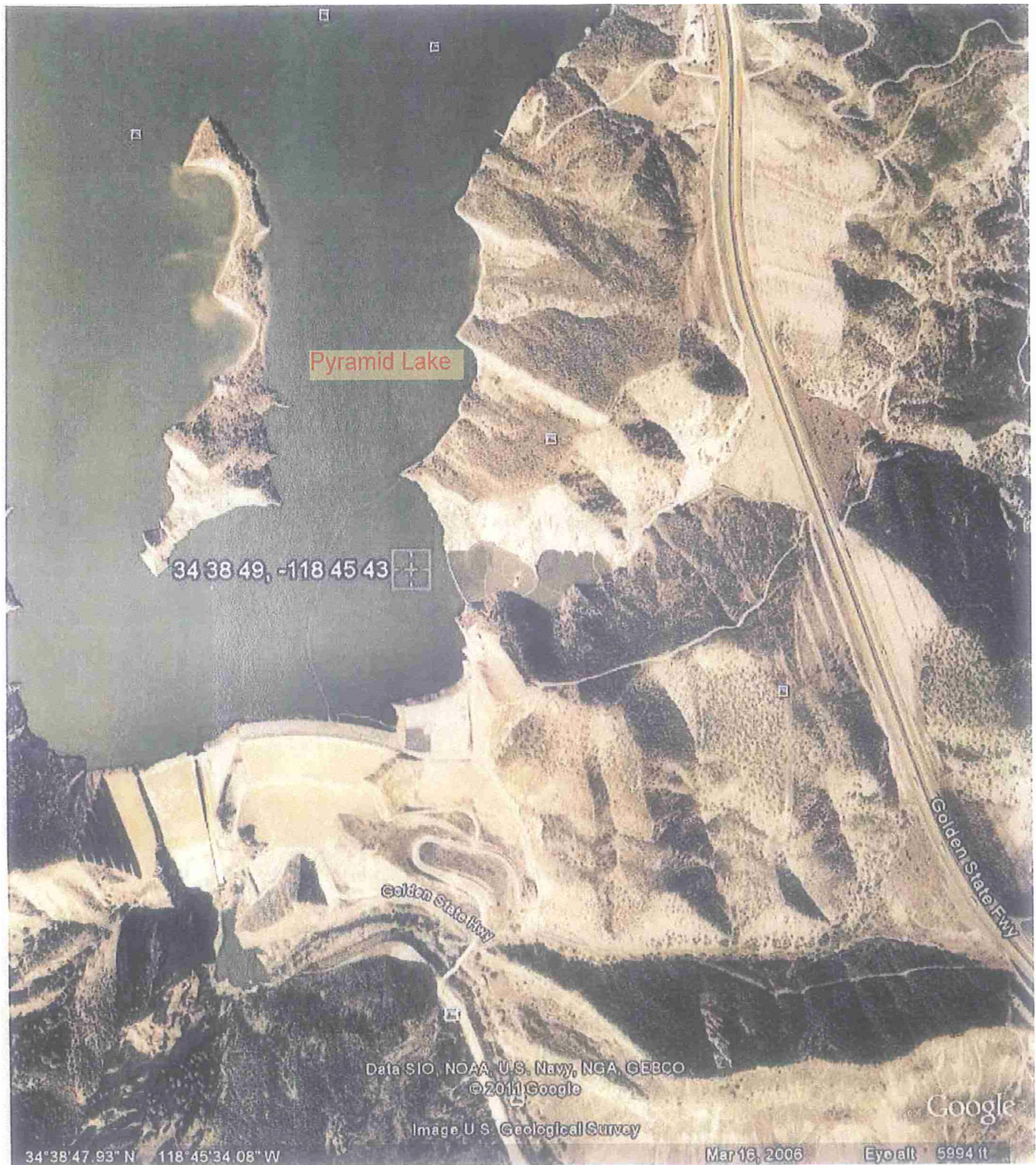
Aerial view of Pyramid Lake and Discharge Point S001 with approximate coordinates.
