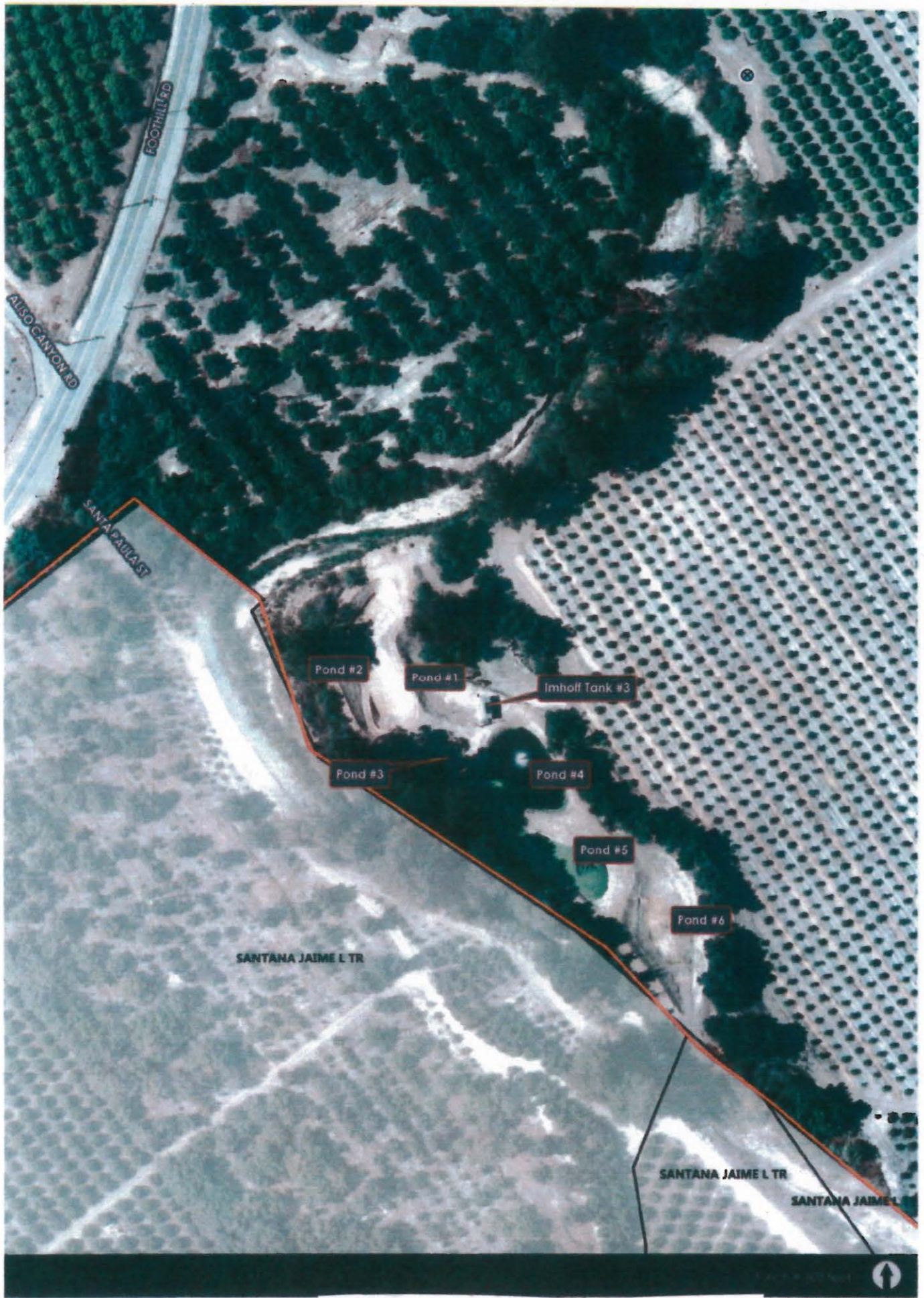
Figure 7. Oliveland Ranch Wastewater Treatment System
