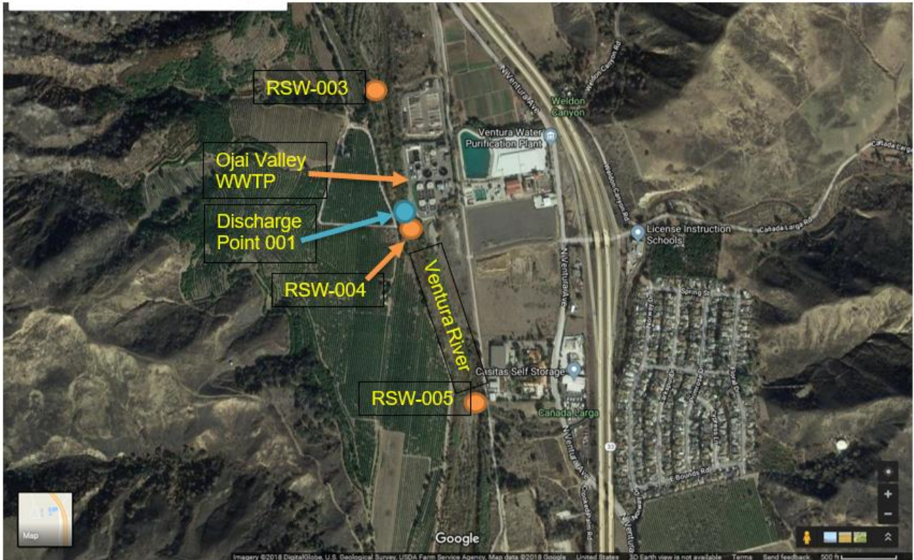
Figure E-1. Ojai Valley WWTP Receiving Water Stations
