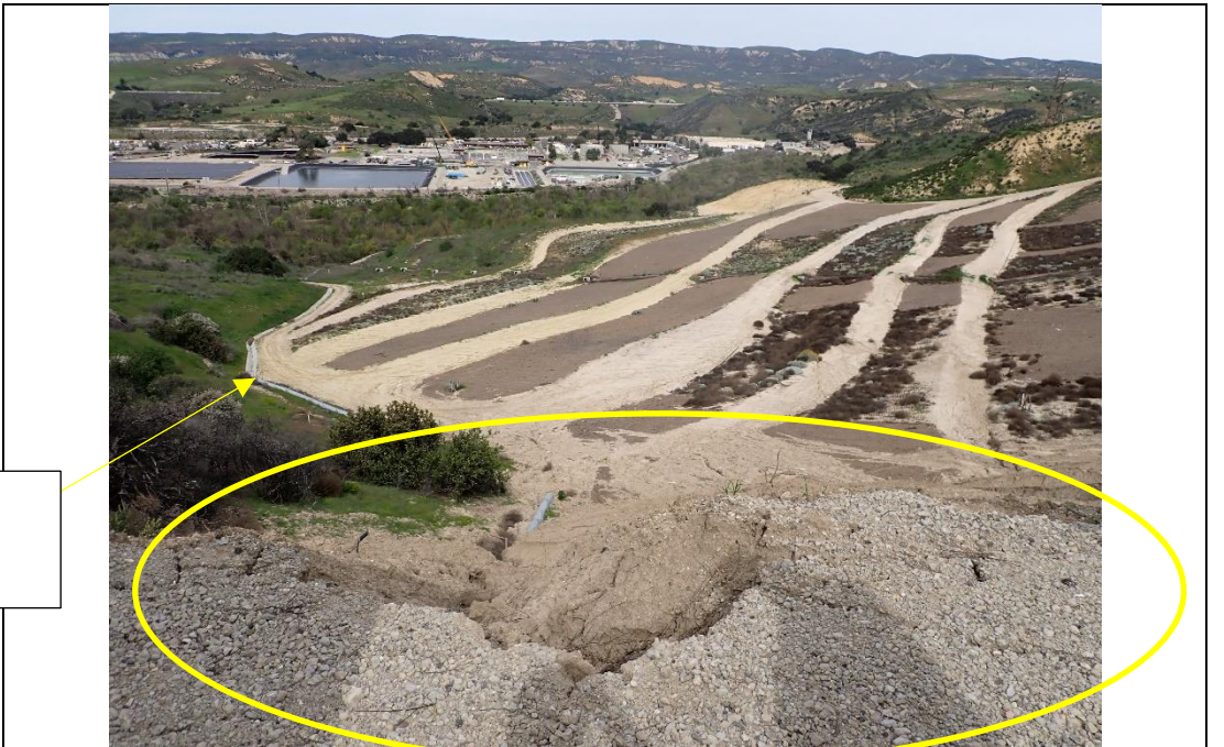
Photograph 2 Pad Cracking / Eroding – Landfill Below and Drainage Pipe
