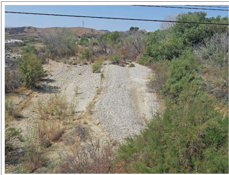
August 25, 2016. View of Castaic Creek Downstream of The Old Road Bridge.
