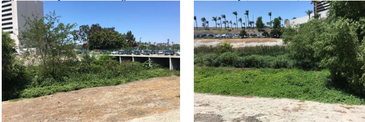
Figure 3. Compton Creek – Vegetation and Sediment Buildup (Downstream)
