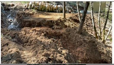
Photo Description: Mound of fill with excavator tracks blocking watercourse channel.
