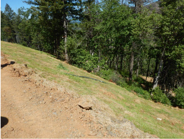
Photo 19: View looking west at an older landslide P8.
