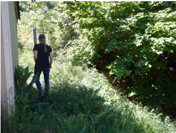
Photo 35: Outlet of culverted watercourse crossing downslope of P11.
