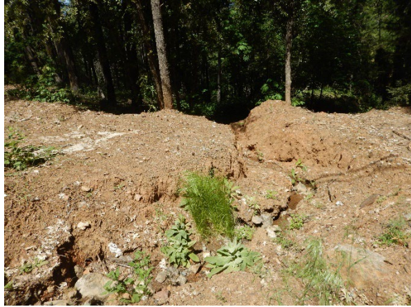
Photo 14: Looking down slope at the channelization of watercourse P5.
