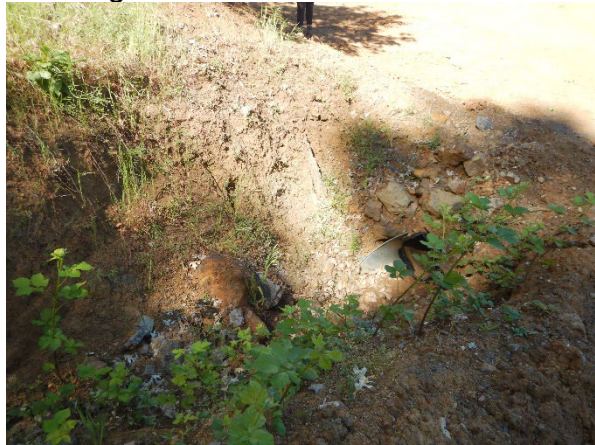
Photo 34: View of inlet of culverted crossing at watercourse P11.
