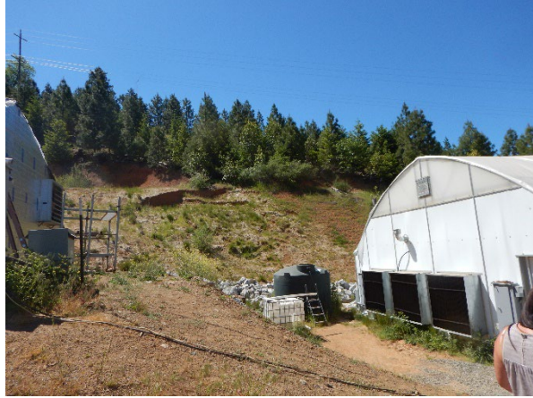
Photo 32: View of upper landslide P10 located above greenhouses.
