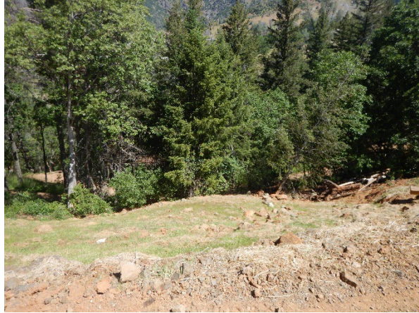
Photo 20: View looking downslope at older landslide P8.
