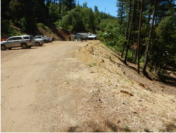
Photo 1: Main parking area and within graded area A1.
