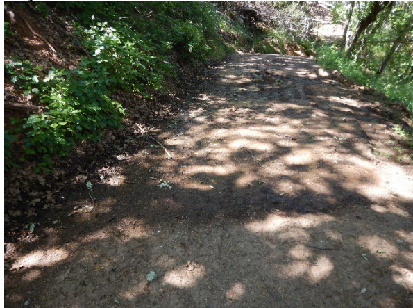
Photo 22: Water flowing across road adjacent to toe of landslide P8.
