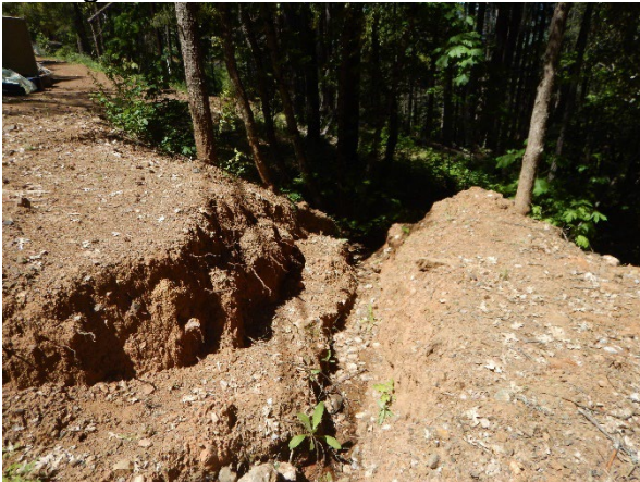
Photo 15: Channel of watercourse P5 through loose fill within A1.
