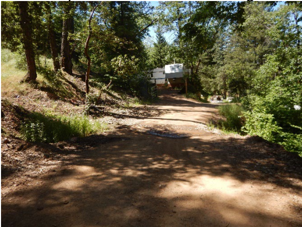
Photo 3: P2 within A1, looking at undeveloped watercourse crossing.
