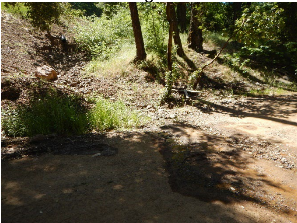
Photo 5: Closer view of undeveloped watercourse crossing at P2 within A1.
