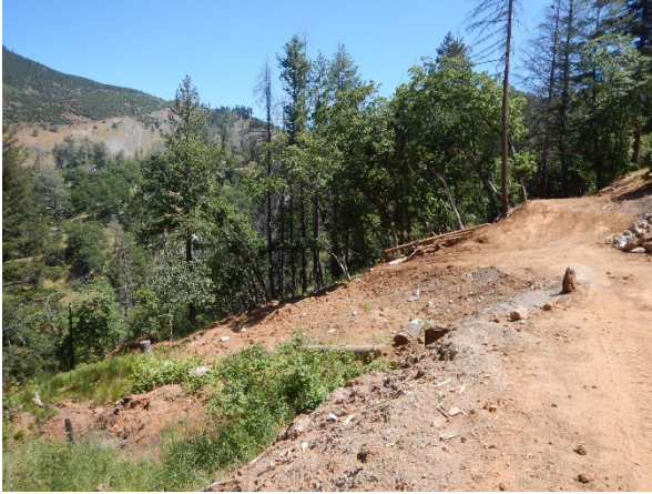
Photo 31: Looking downslope at lower landslide P10 slide mass.
