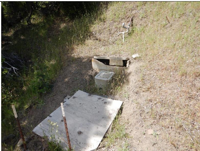
Photo 21: Water diversion structure at WQ13
