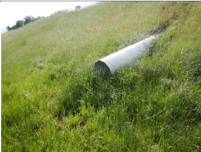
Photo 29: Outlet of a watercourse crossing culvert at WQ19
