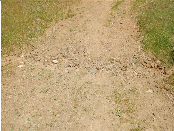
Photo 9: Rocked fill stream crossing at WQ6
