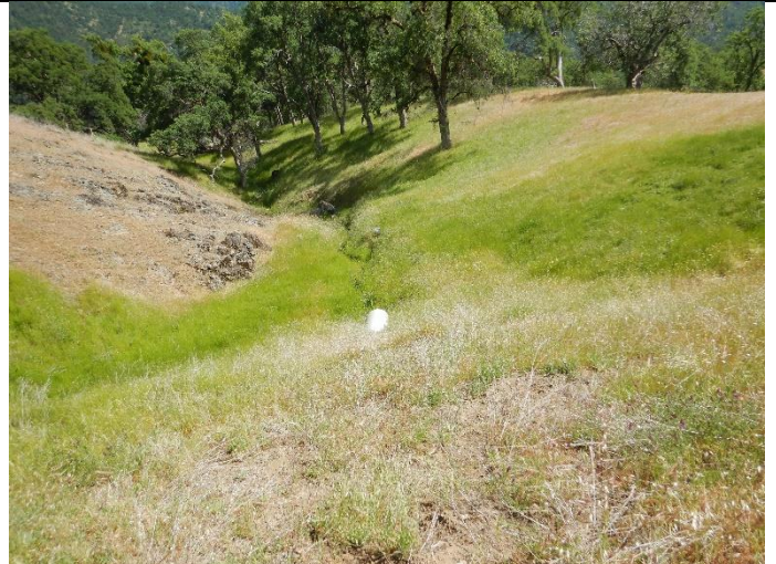
Photo 20: Outlet of a culverted watercourse crossing at WQ12
