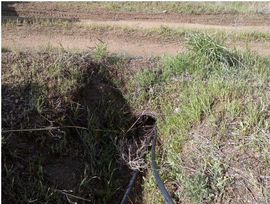
Figure 9—Looking southwest at a ten-inch diameter culverted watercourse crossing at WQ4. The watercourse upstream and to the back of the photographer is approximately three-feet wide.
