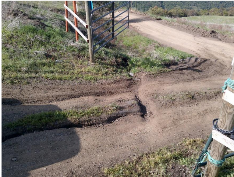
Figure 5—Looking southwest across the gated access to the Property at WQ1. Ruts have eroded into the road-surface.
