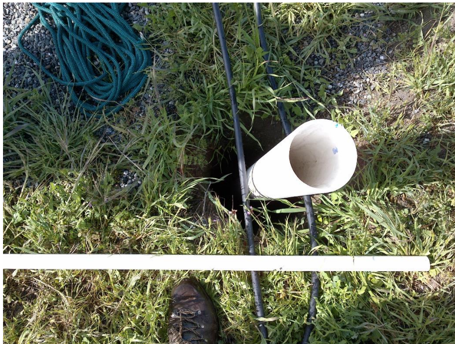
Figure 7—Looking down at a four-inch diameter plastic pipe in a twelve-inch diameter hole at WQ2. The well hole does not have a casing or cap to protect groundwater from any pollutants that could be introduced at the surface.
