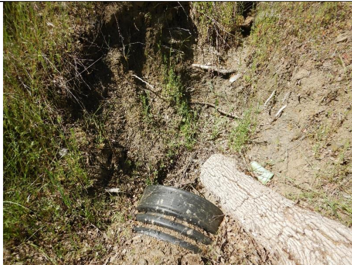
Photo 15: Inlet of a culverted watercourse crossing at WQ11
