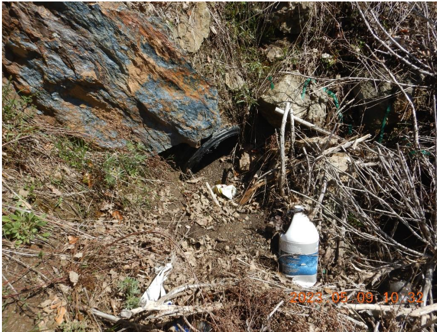
Figure 18—Partially buried culvert outlet at WQ6 among cultivation waste including plant stalks and plastic containers.
