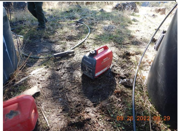
Photo 22 – uncontained generator and gasoline tank at WQ4
