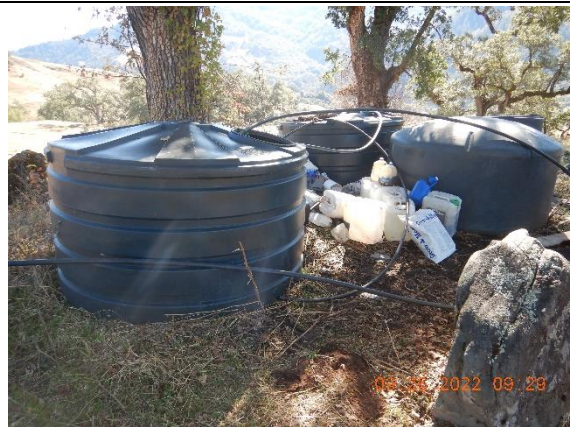
Photo 34 – water storage tanks at inspection point WQ4
