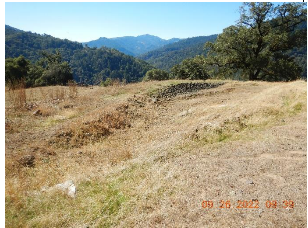
Photo 4 – Dry onstream pond at inspection point WQ5 without any engineered outflow
