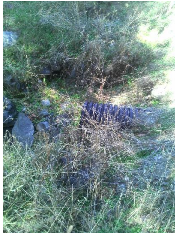
Photo 17 – Properly functioning culvert outlet at inspection point WQ31
