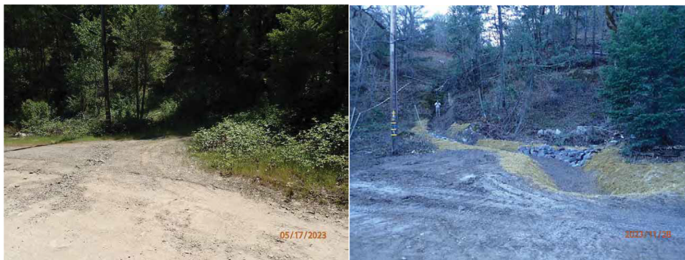
Left: Pre-implementation – View from the left outboard edge of the road looking upslope toward the utility pole located near the natural channel alignment. Right: Post-implementation – View from the left outboard edge of the road looking upslope at the new channel alignment.
