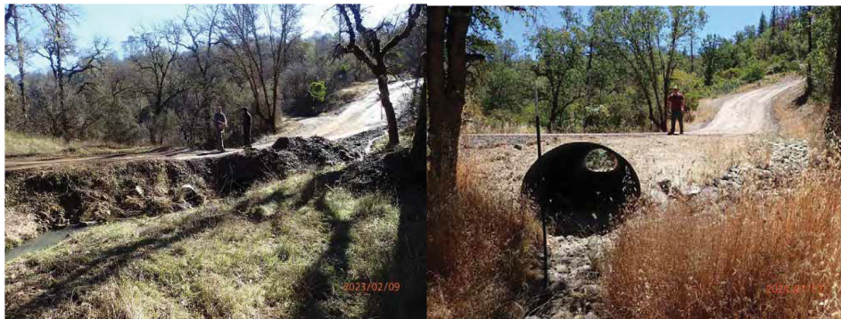
Left: Pre-implementation - View from upstream of the crossing looking downstream toward the old culvert inlets. Right: Post-implementation – View from upstream of the crossing looking downstream toward the new culvert inlet.
