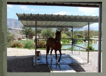
Cover wash areas- make sure drains are connected to sewer.
