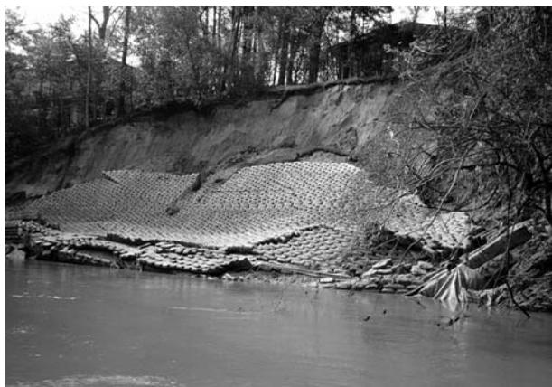
**Figure 3.** Failure of sacrete bank erosion control structure because of high pore-water pressure in the bank behind the structure. Photograph: Joan L. Florsheim.
