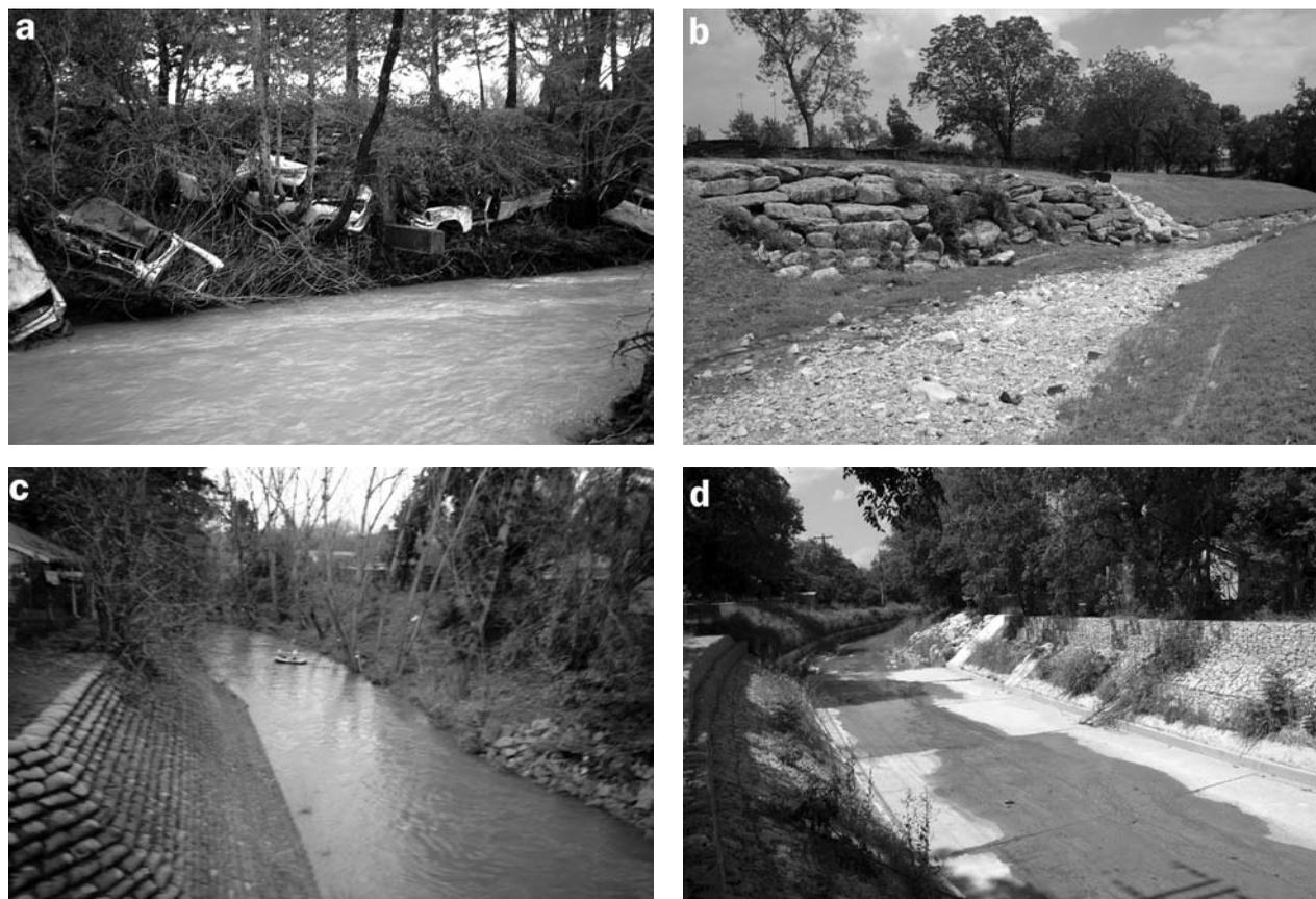
**Figure 2.** Examples of channel bank structures. Some bank erosion-control structures are not designed or engineered; rather, they are ad hoc attempts to prevent local land loss or damage. (a) Car bodies; (b) riprap; (c) sacrete on left bank, riprap on right bank; and (d) rock-filled gabions along banks of concrete-lined channel. Photographs: Joan L. Florsheim (2a and 2c) and Anne Chin (2b and 2d).
