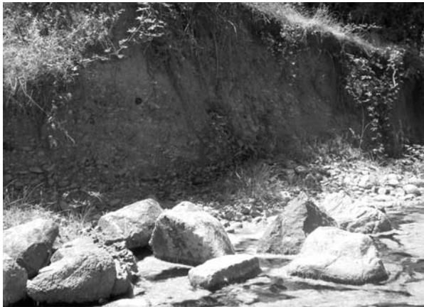
**Figure 4.** Bank erosion processes continuing behind large rock riprap originally placed at the base of the bank. If left isolated in the channel, riprap may become an impediment to future restoration. Photograph: Joan L. Florsheim.
