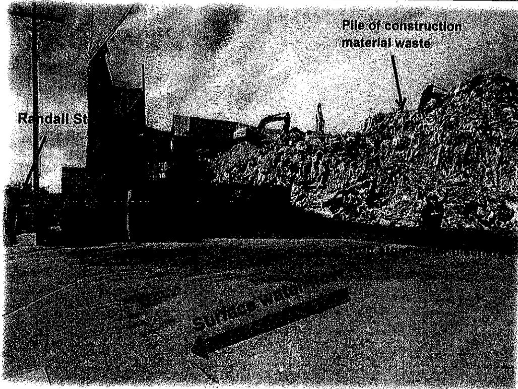
Photo 2 – Standing on Randall Street, facing west. A large pile of construction material waste located as close as about 80 feet away from Randall Street. Evidence of non-stormwater discharge onto Randall Street was observed.
