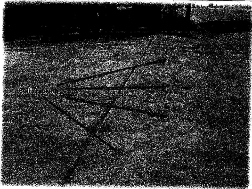
Photo 4 – Same position as photo number 3, showing non-stormwater discharge and soil tracking onto Pendleton Street.
