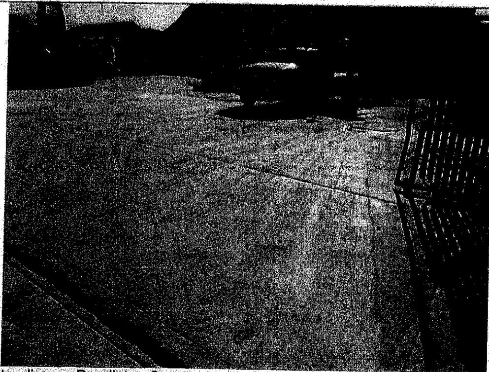
Photo 1 – Standing on Pendleton Street, outside Exit/Entrance 1, facing east. Sediment track-off is observed from the Site onto the Pendleton Street.
