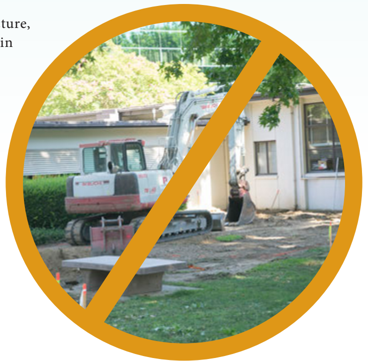
Figure V-1. Keep heavy equipment off areas intended for infiltration
