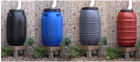
Figure 1. Aboveground storage (Porter County IN)
