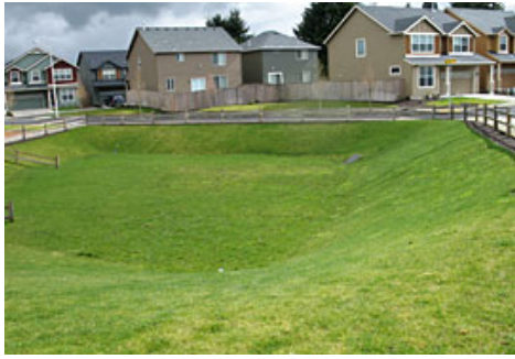
Figure 1. Detention basin (Stormwater Partners SW Washington)
