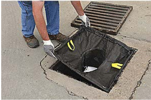
Figure 1. Drain inlet insert (Grainger)
