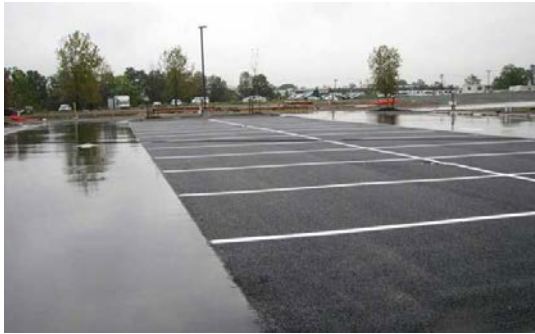
Figure 1. Porous pavement (EPA)
