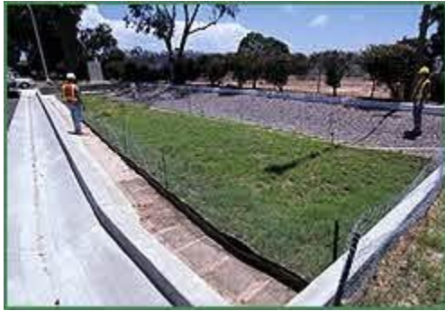
Figure 1. Vegetated Buffer Strip (Caltrans)
