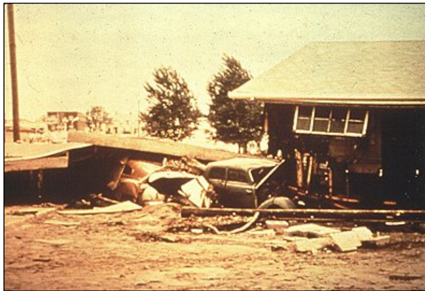
Photograph RO-1—Devastating flooding from the South Platte River in 1965 emphasizes the importance of accurate flood flow projections.
