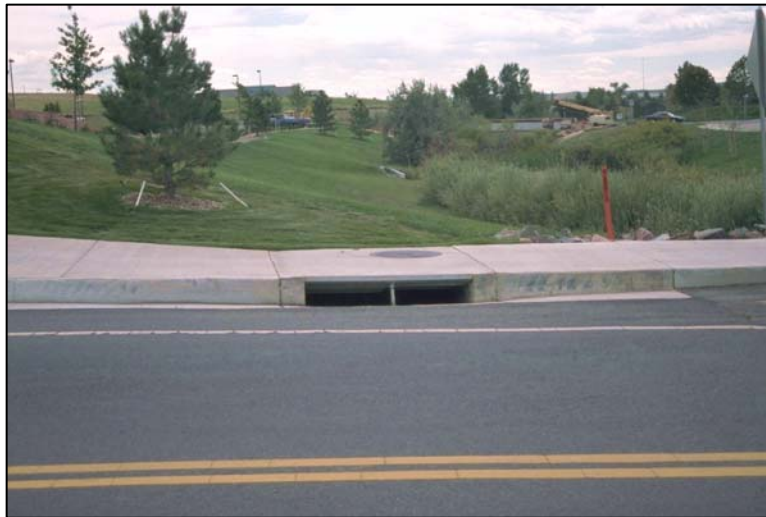
Photograph ST-4—Inlets that are located in street sags and sumped can be highly efficient.
