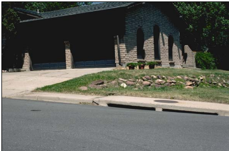
Photograph ST-3—Gutter/street slope is a major design factor for both street and inlet capacity.
