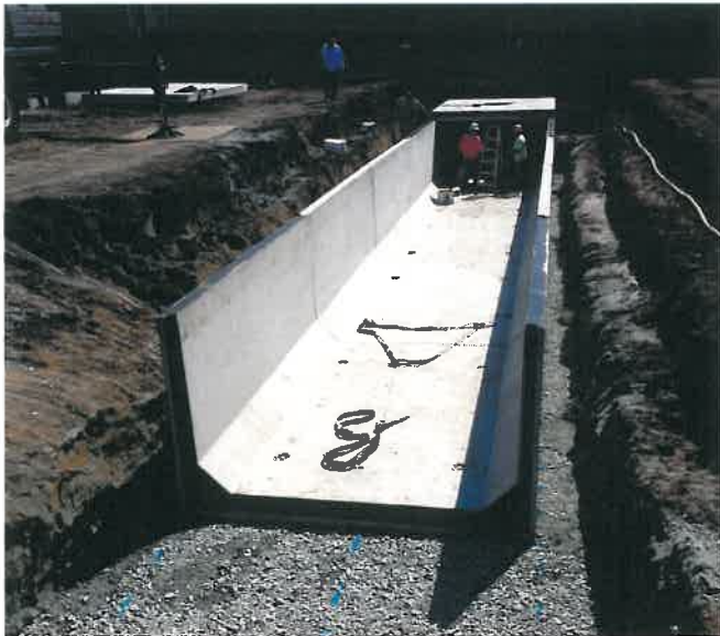
Fig. C-3: Installing precast concrete vault sections
