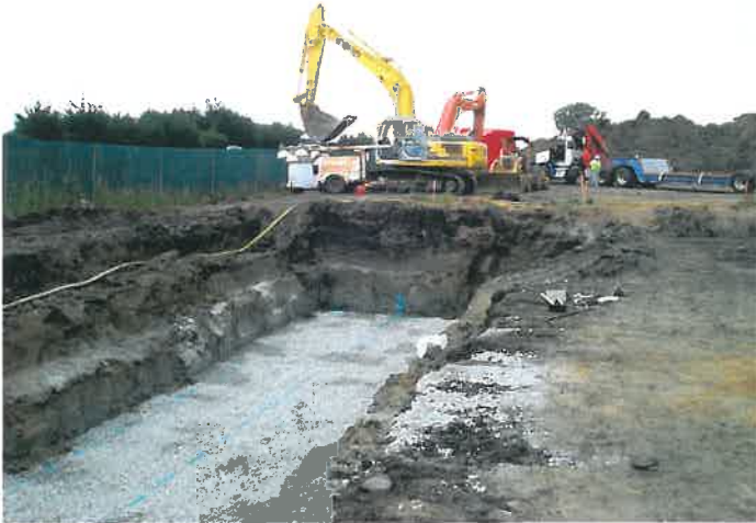
Fig. C-1: Excavation and subbase preparation
