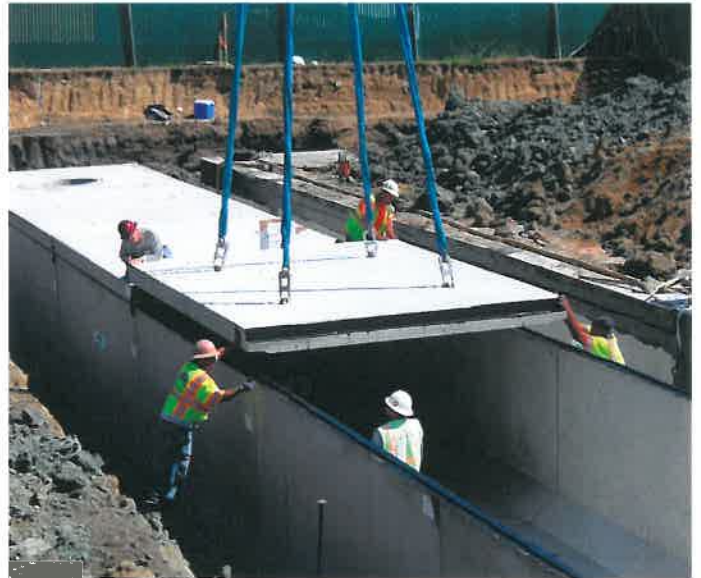
Fig. C-4: Installing precast roof slab
