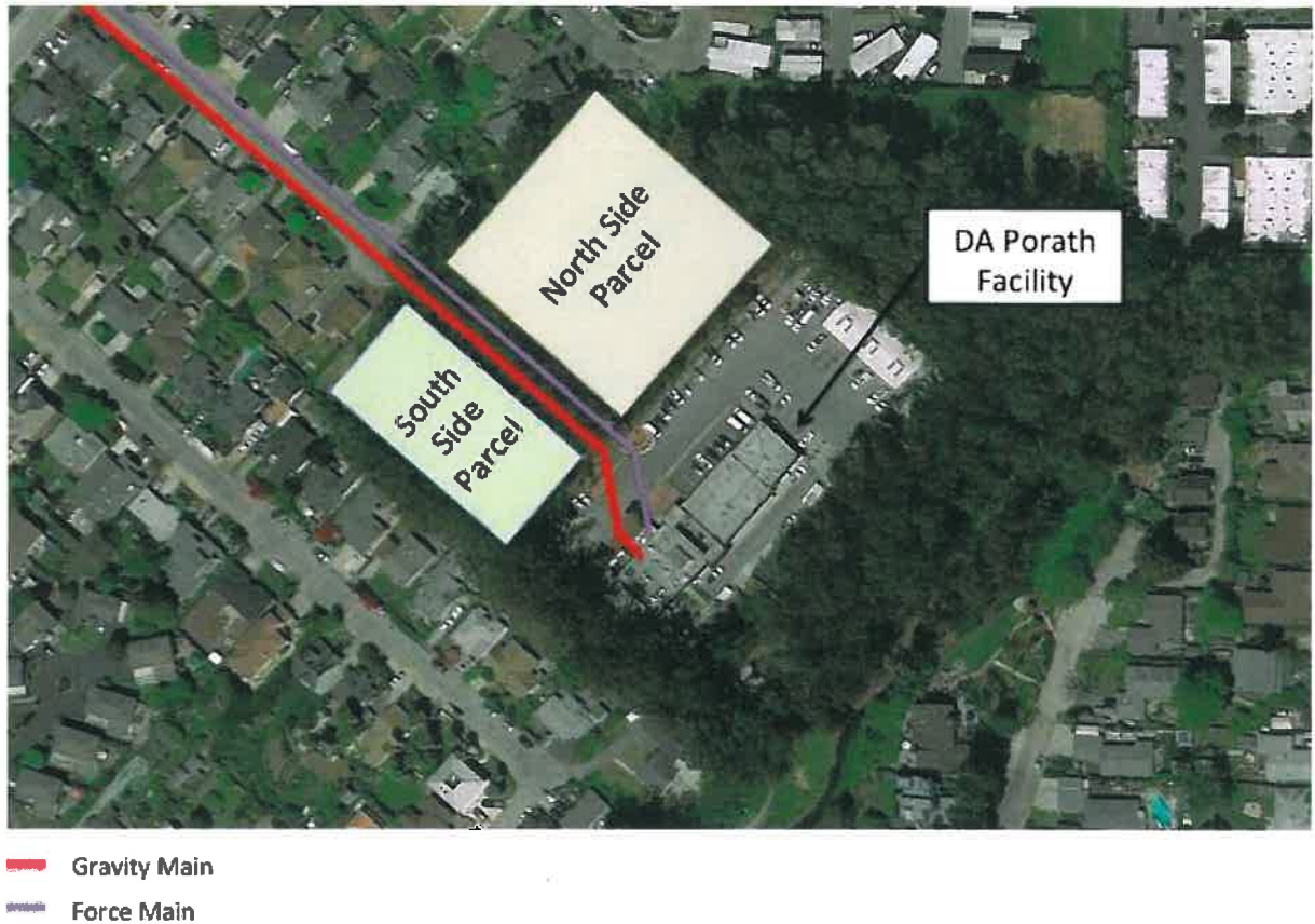
Figure 1 Site Aerial View
