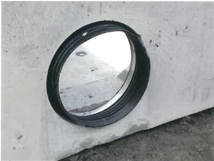
Fig. C-5: Sewer pipe boot at pipe connection
