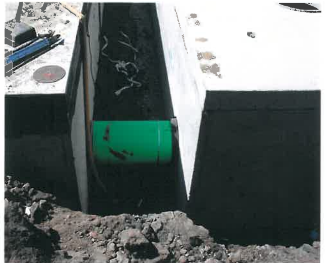
Fig. C-6: Piping connection between chambers
