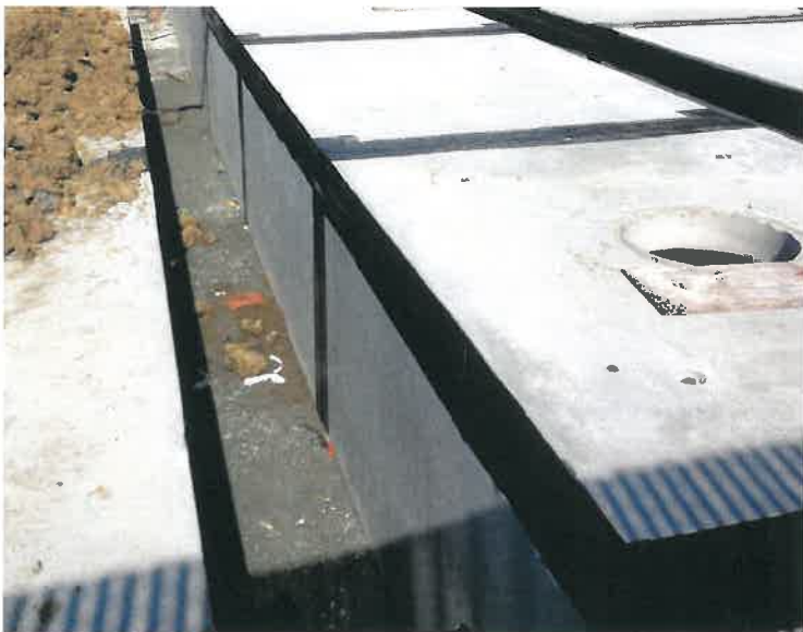
Fig. C-7: Sealants to assure water tightness of vaults
