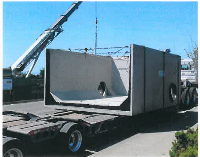
Fig. C-2: Vault sections arriving at project site
