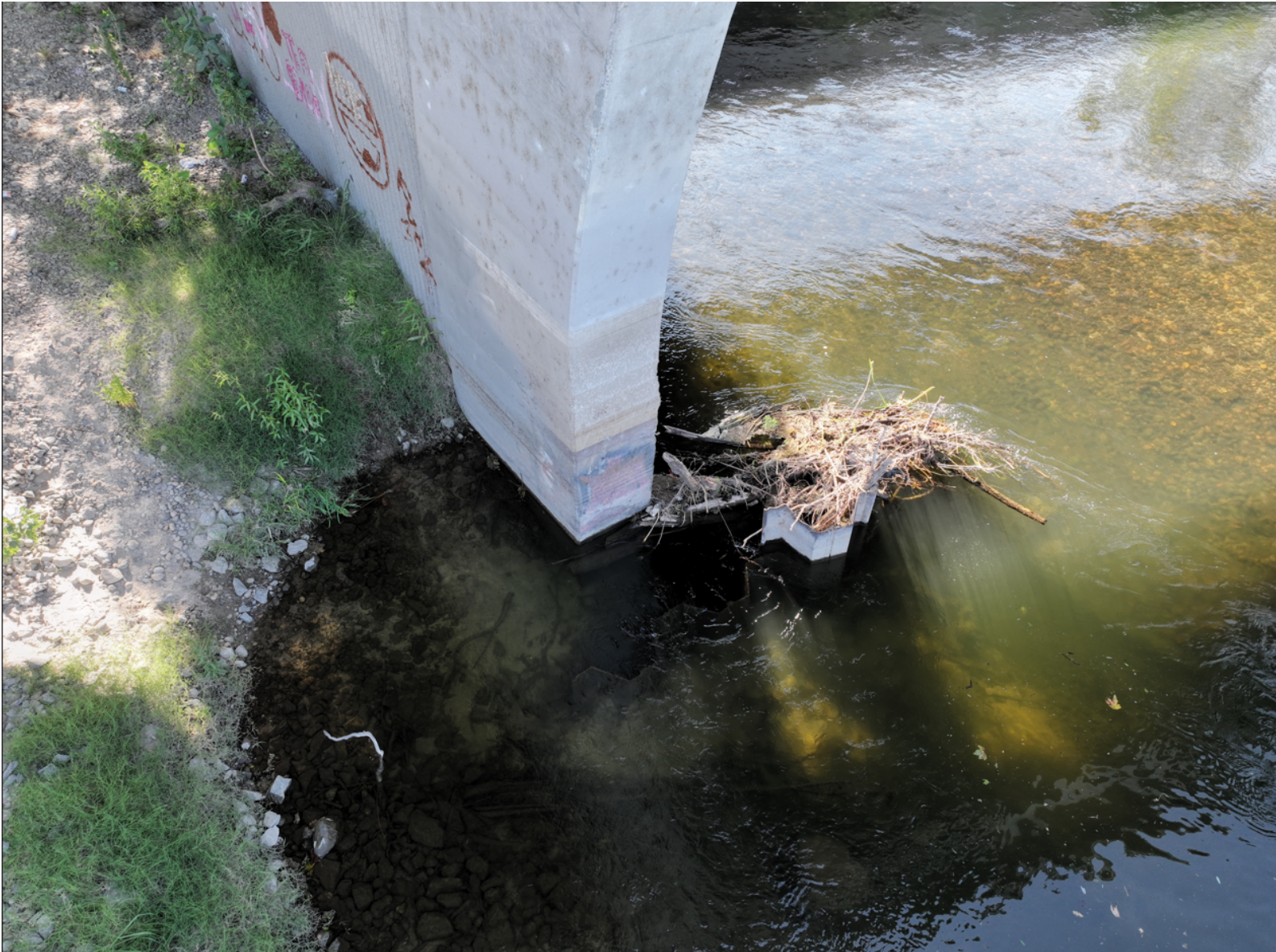
Figure 1: Sheet pile to be removed
