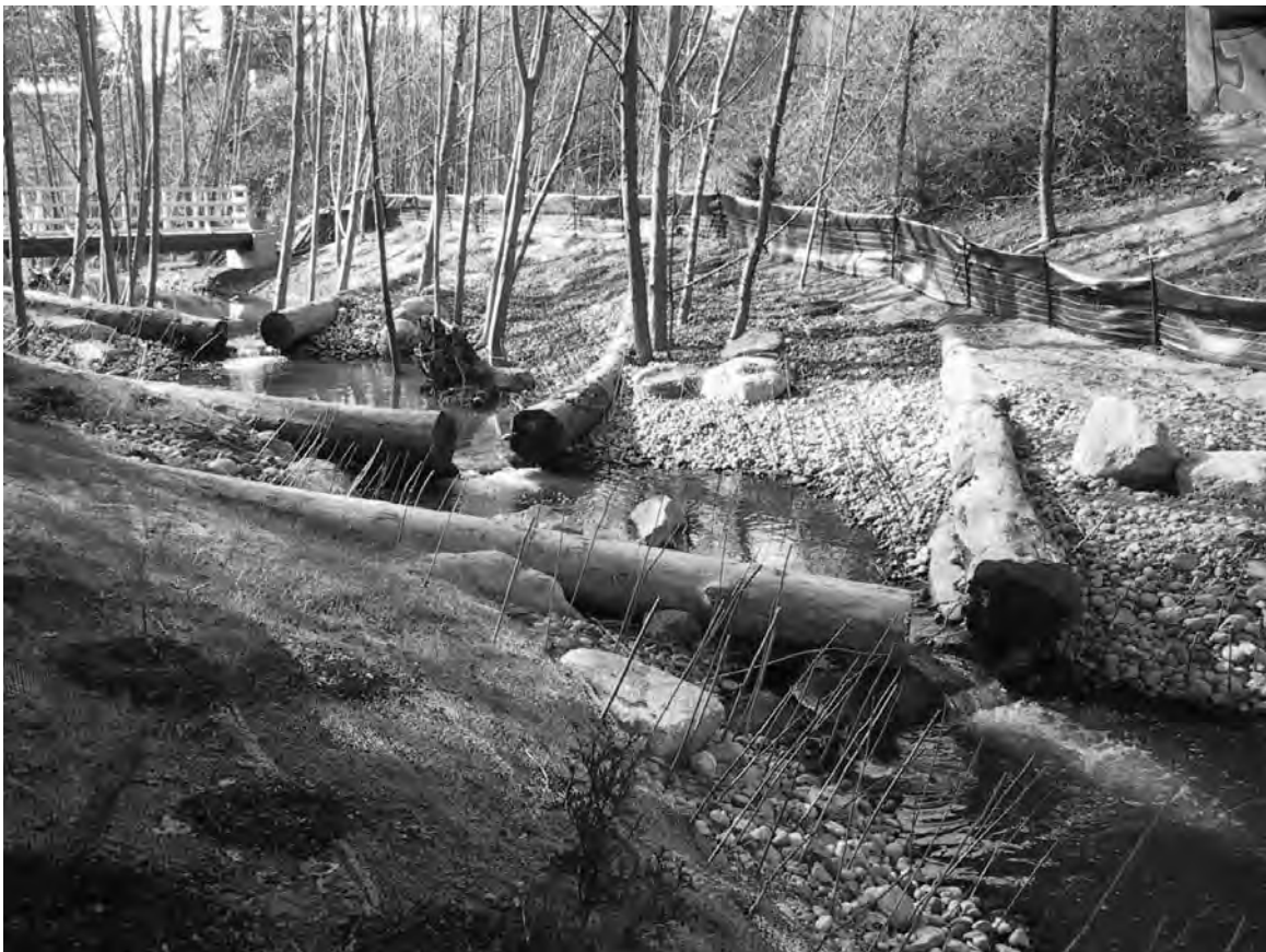
FIG. 4. Longfellow Creek, in the city of Seattle, Washington, shortly after channel reconstruction with log deflectors, imported channel-bed sediment, and riparian plantings.
