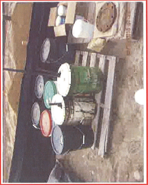
Failure to cover and provide secondary containment.
