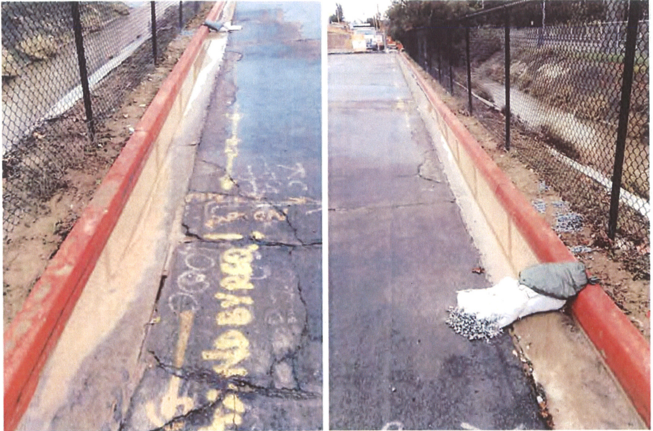
Photos 2 & 3. Ponded Water at First Set of Gravel Bags Downstream of Akins Avenue Entrance/Exit (Looking downstream and upstream, respectively)
