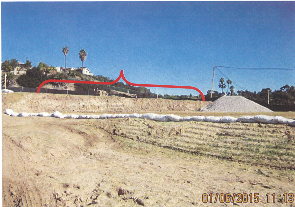
Photo 5. Sidewall without adequate erosion control
