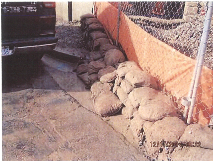
Photo 1. Evidence of sediment discharge at Akins entrance/exit
