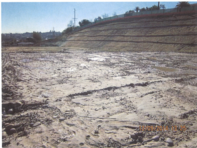
Photo 1. Lot lacking erosion control BMPs
