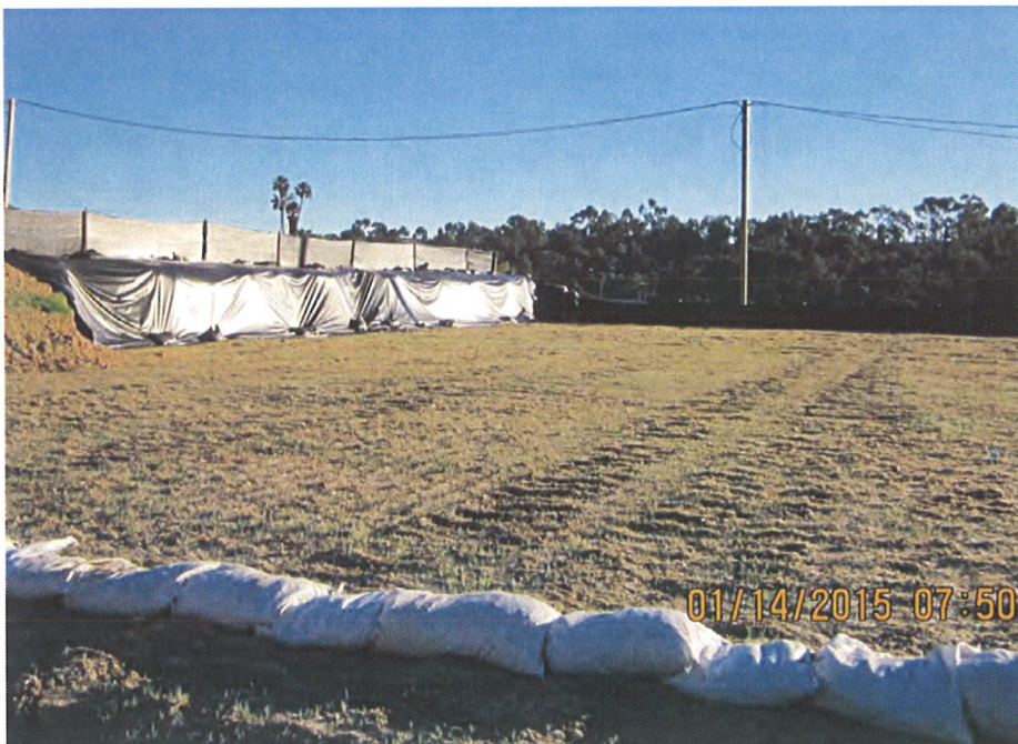
Photo 6 Sidewall protected with plastic sheeting.
