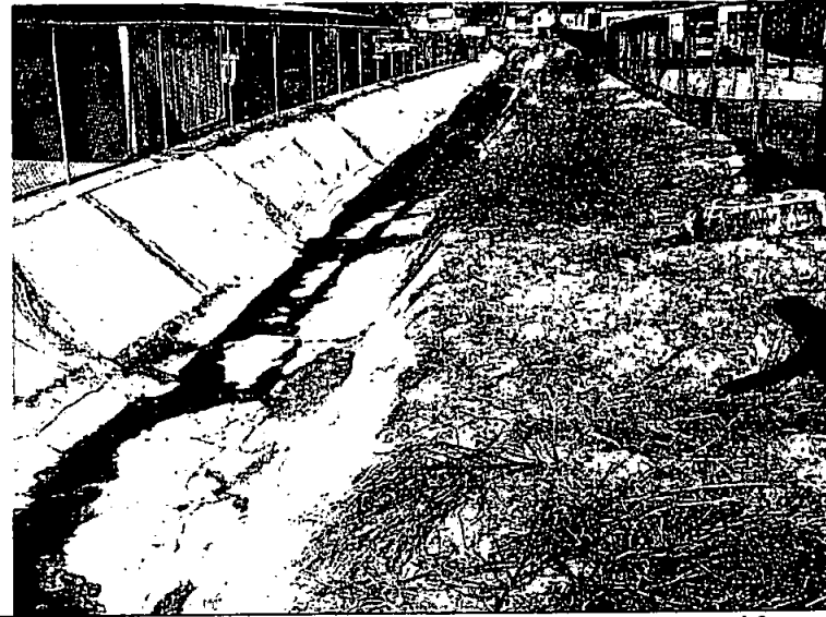
Drainage looking downstream (north) after vegetation removal from pilot channel construction (2/14/13)
