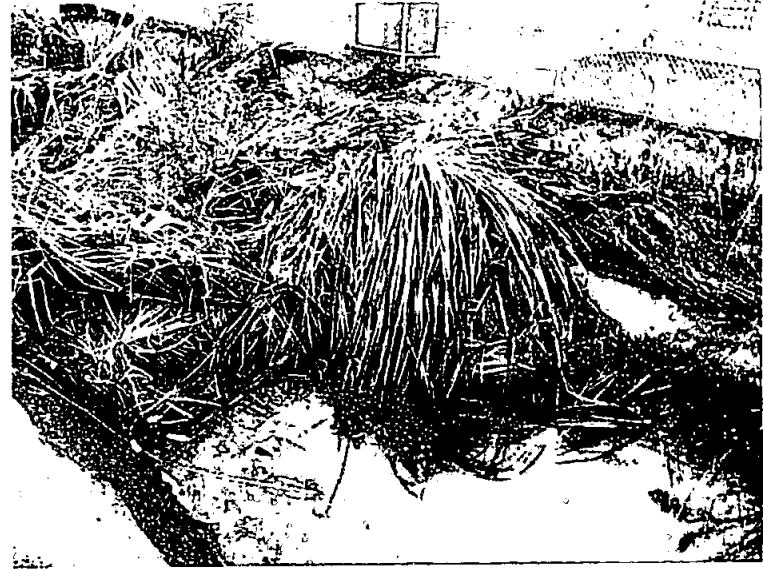
Remaining vegetation (that was to remain in the channel) that has floated downstream and has piled up and blocking flow (12/18/12)
