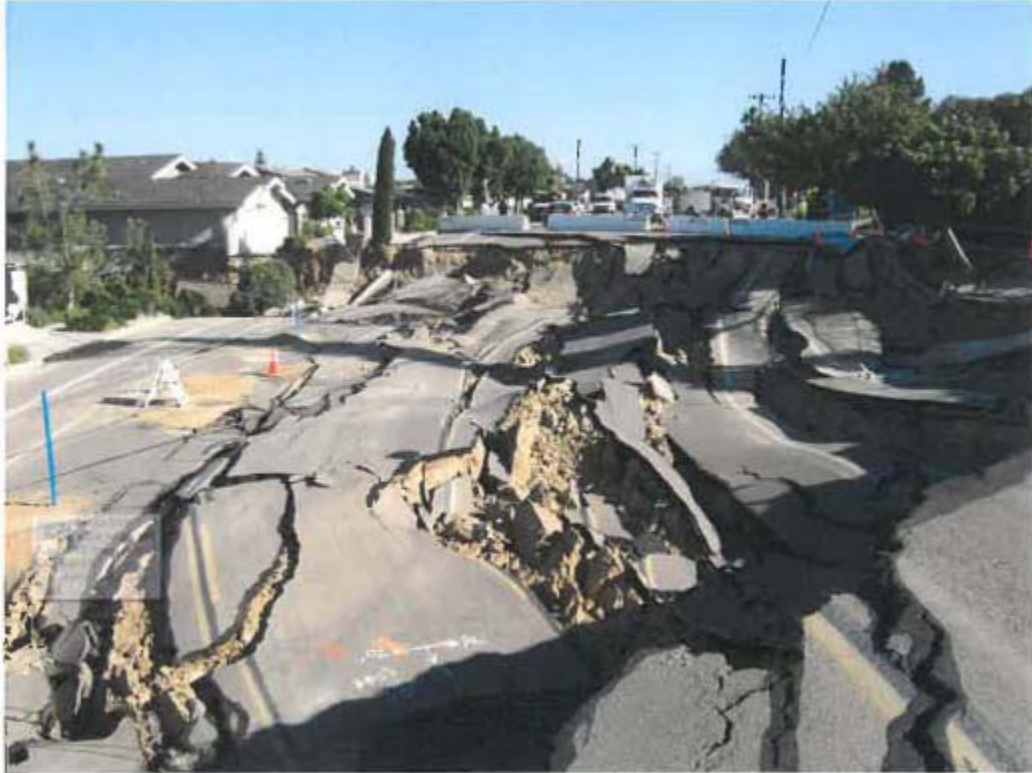
Photo 1 – La Jolla Landslide (Ardath Shale Formation, Claystone, Hydrologic Group D)
