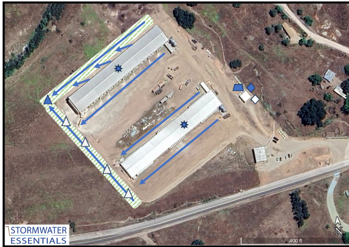
Figure 4. Map Showing Location of the Pullet Farm Structures and Surface Runoff Direction
