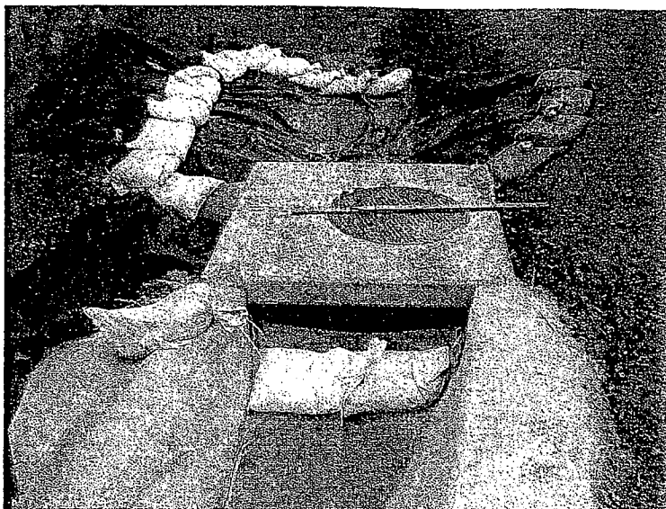
Photo 35 Inlet with gravel bag protection. NOV photo 38.
