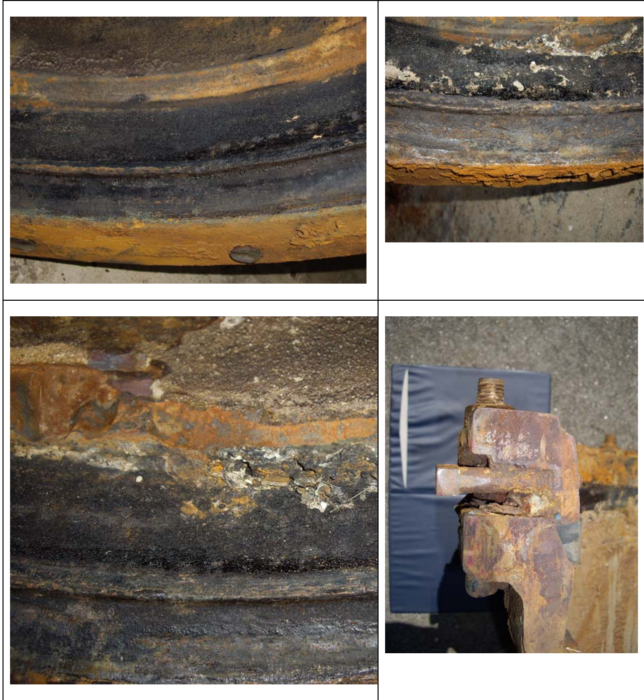
Figure 6 – Four photos showing asphaltic coating and joint condition
