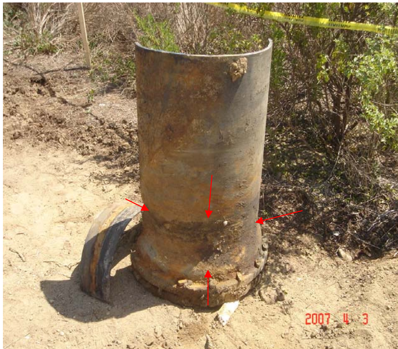
Figure 3 – Sectioned pipe opposite side of failure (above springline)
