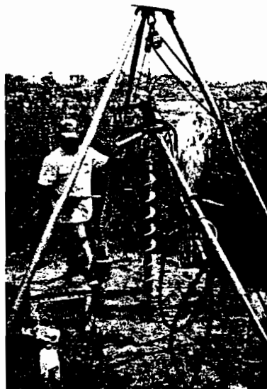
Sediment sampling with tripod drill
